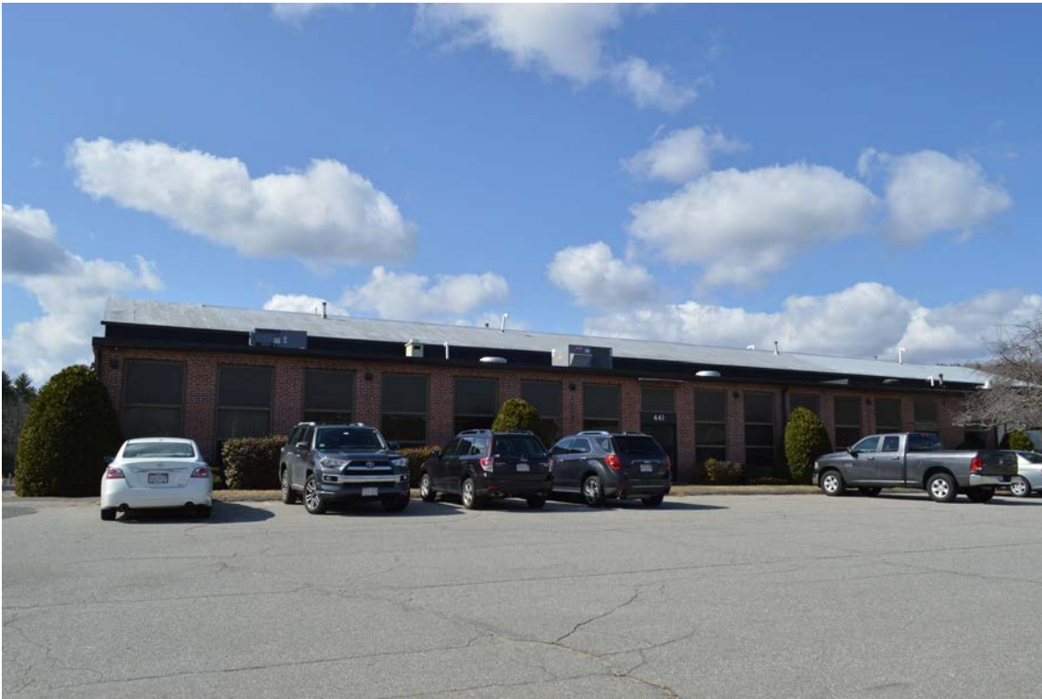
Photo 16. 441 Main Street (STU.117), looking southwest.
