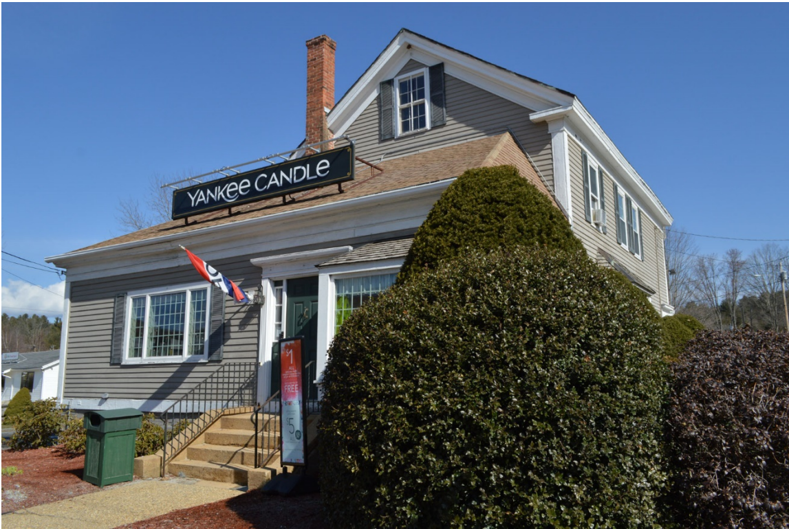
Photo 14. 434 Main Street (STU.92), looking northwest.
