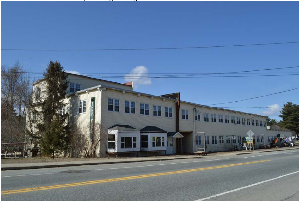
Photo 13. 433 Main Street (STU.118), looking northwest.
