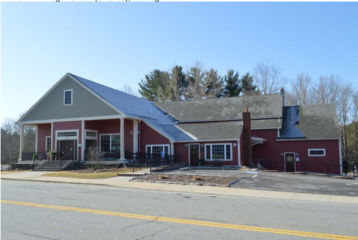
Photo 5. 419 Main Street (STU.122), looking southeast.
