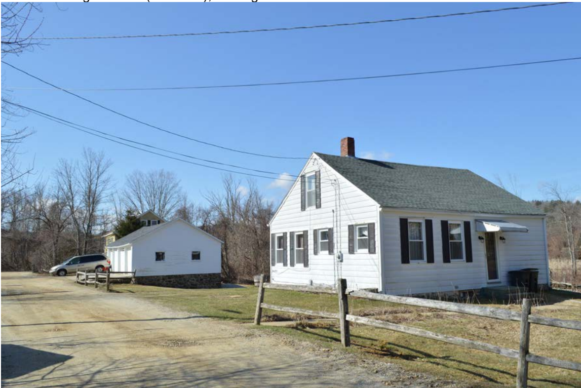
Photo 3. 7 Auger Street (STU.100) and Garage, looking southwest.
