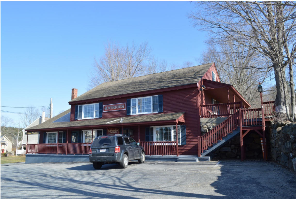
Photo 12. 426 Main Street (STU.90), looking northwest.
