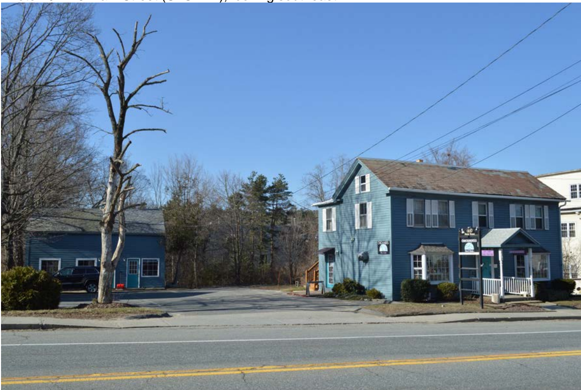
Photo 11. 425 Main Street (STU.120), looking northwest.
