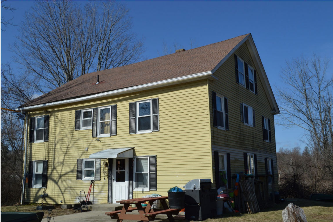
Photo 2. 3 Auger Street (STU.101), looking southwest.
