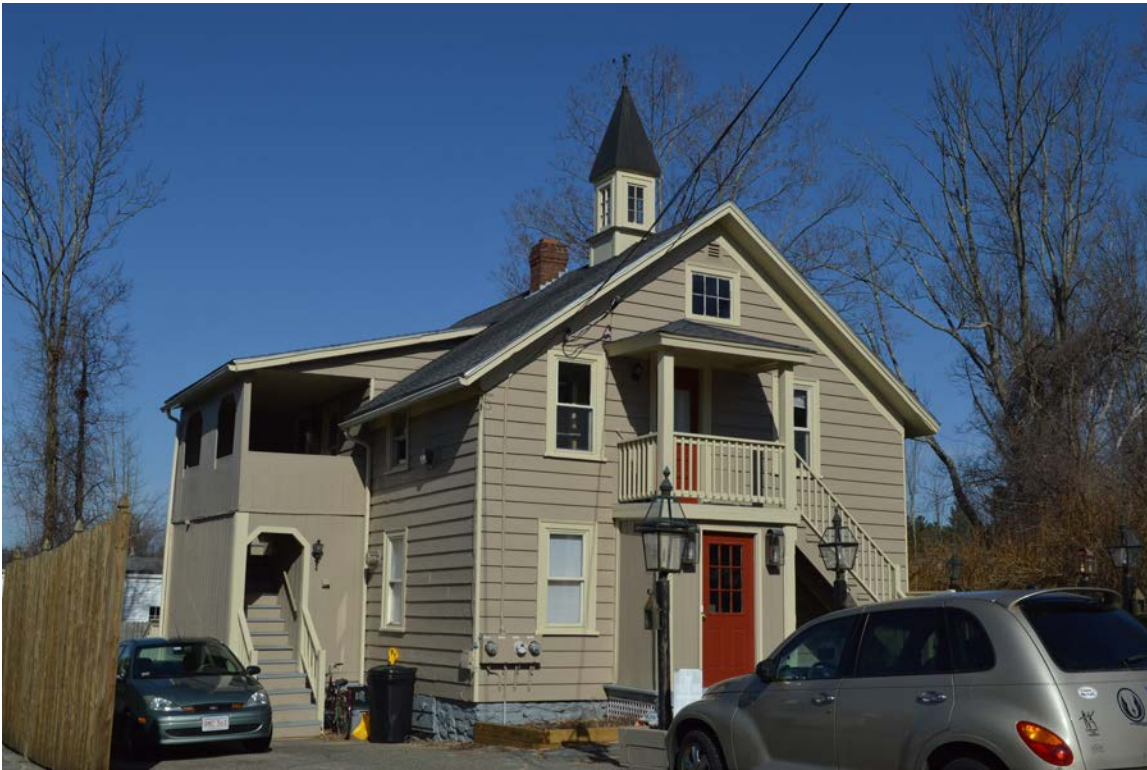
Photo 22. 5 Snell Street (STU.94), looking northwest.
