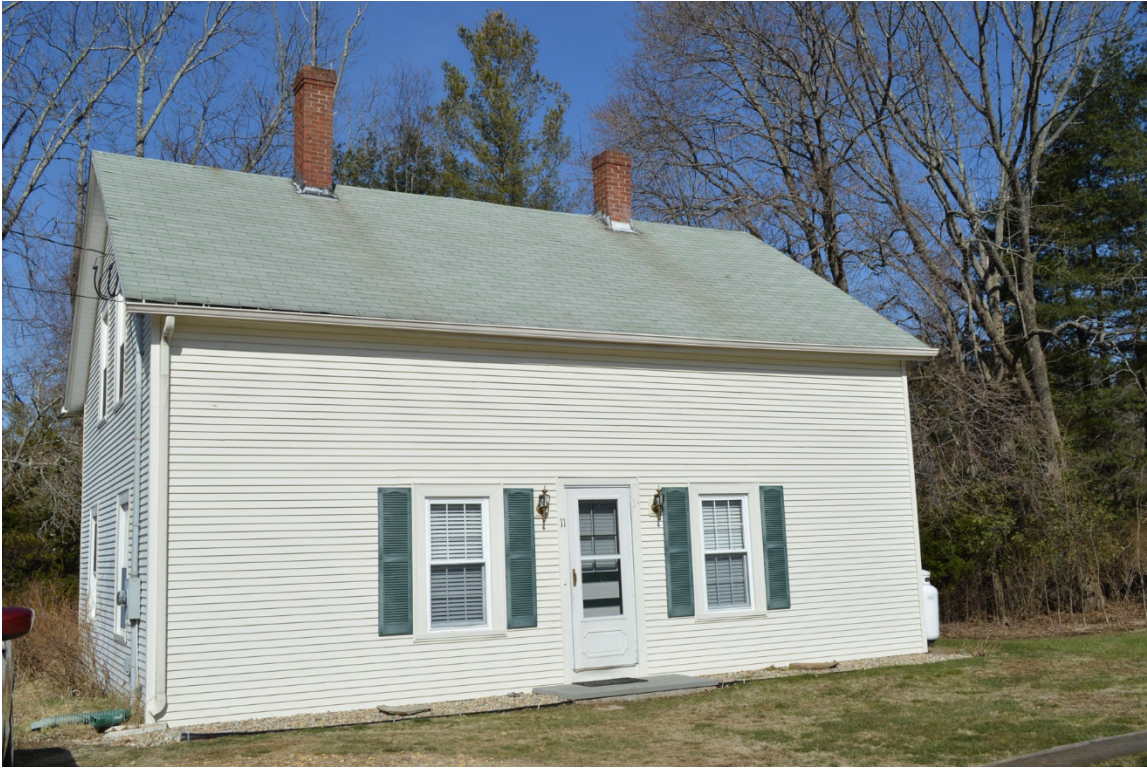
Photo 4. 11 Auger Street (STU.99), looking northwest.
