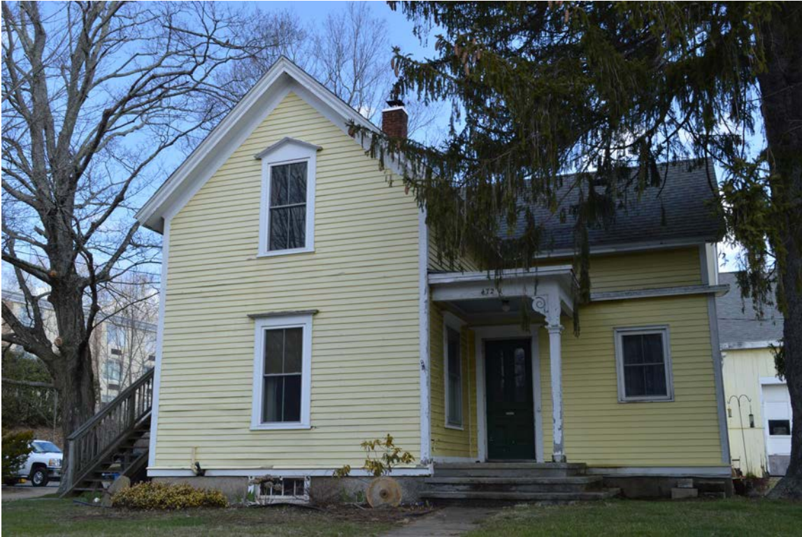
Photo 18. 472 Main Street (STU.111), looking northwest.
