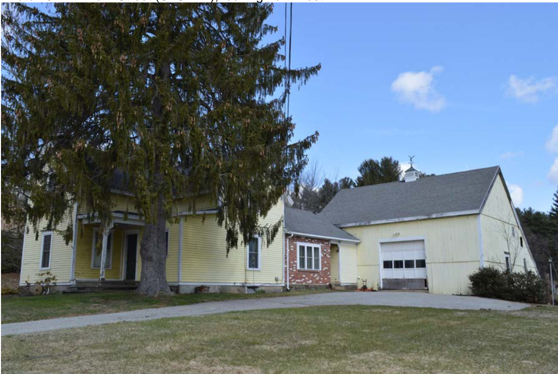
Photo 19. 472 Main Street (STU.111), looking northwest.
