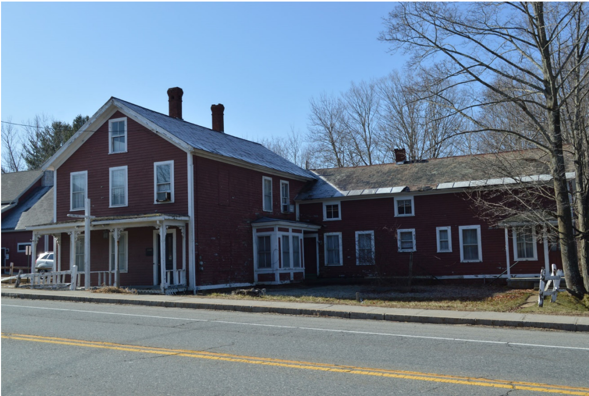
Photo 10. 423 Main Street (STU.121), looking southeast.
