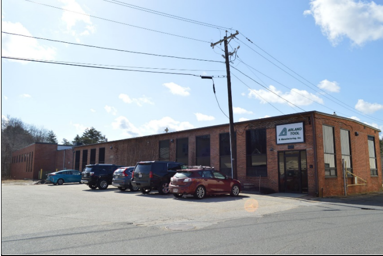
Photo 1. 421 Main Street (STU.119), looking southwest.
