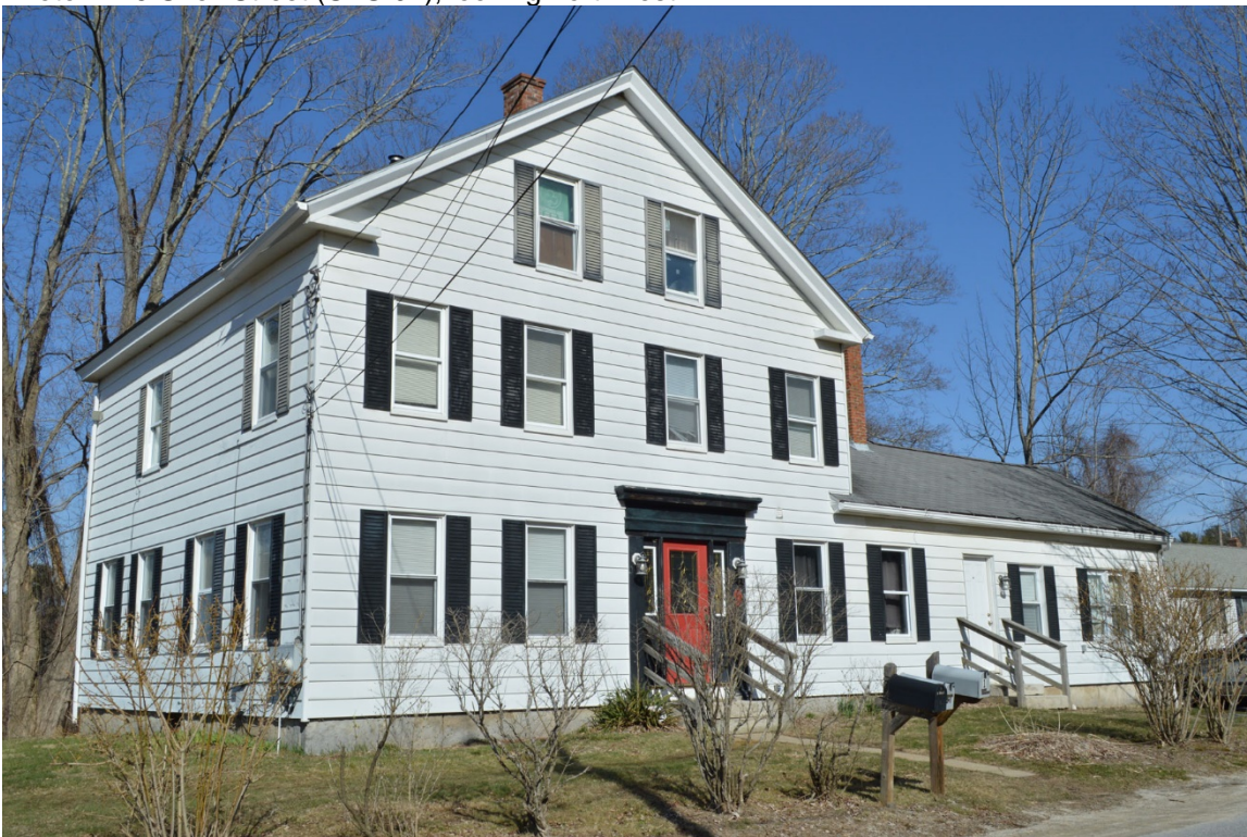
Photo 23. 9 Snell Street (STU.95), looking northwest.
