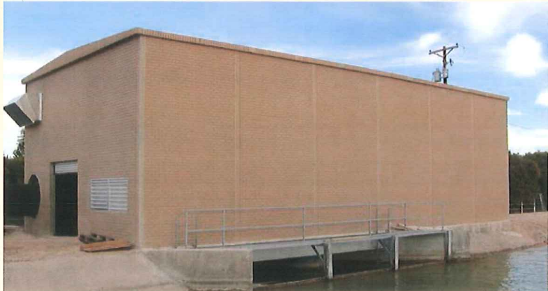
Unobstructed 30' W x 24' H x 60' L space allows room for large hydroturbine equipment, Mesa, AZ
