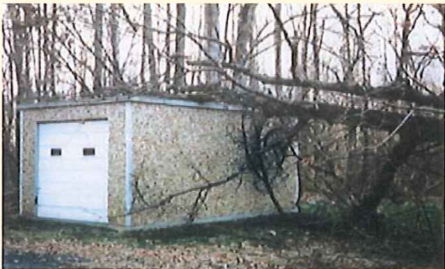
Fallen mature oak tree causes no damage
