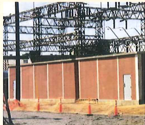
Electrical Substation, Board of Public Utilities
