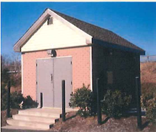
Generator Building, Oliver City Sanitary Sewer System, Warrenton, VA
