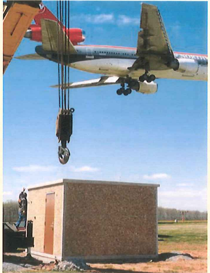
Quick installation of Navigational Aide Building at Dulles International Airport
