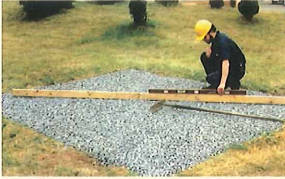
Simple site preparation, no footings required
