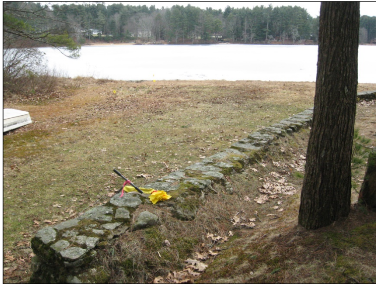
Photograph No. 3: Construction access, facing south.
