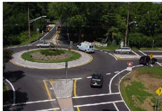
Example of a roundabout from North Haven, New York
