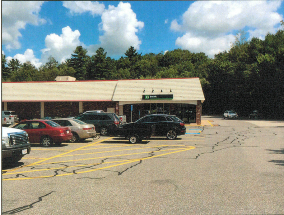
EXISTING SITE PHOTOGRAPH
