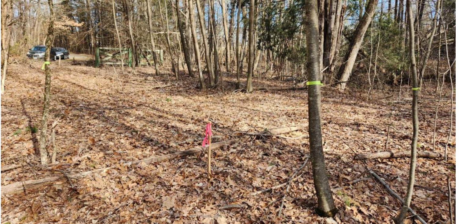
Photo #1: Location of Soil Boring B-1, indicated by wooden stake. B-1 is proposed within the locally regulated 50-ft No Structure Zone, and 100-ft and 200-ft Buffer Zone to BVW. Tree removals are required to create a 20-ft wide cleared path centered on the soil borings. Trees proposed for removal are flagged in yellow flagging. Facing northeast.
