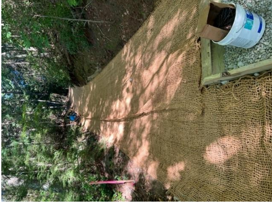
Stabilization fabric installed prior to stone placement
