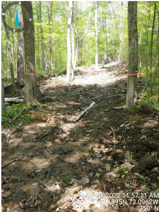
3. Excavated & finish-graded replication area
