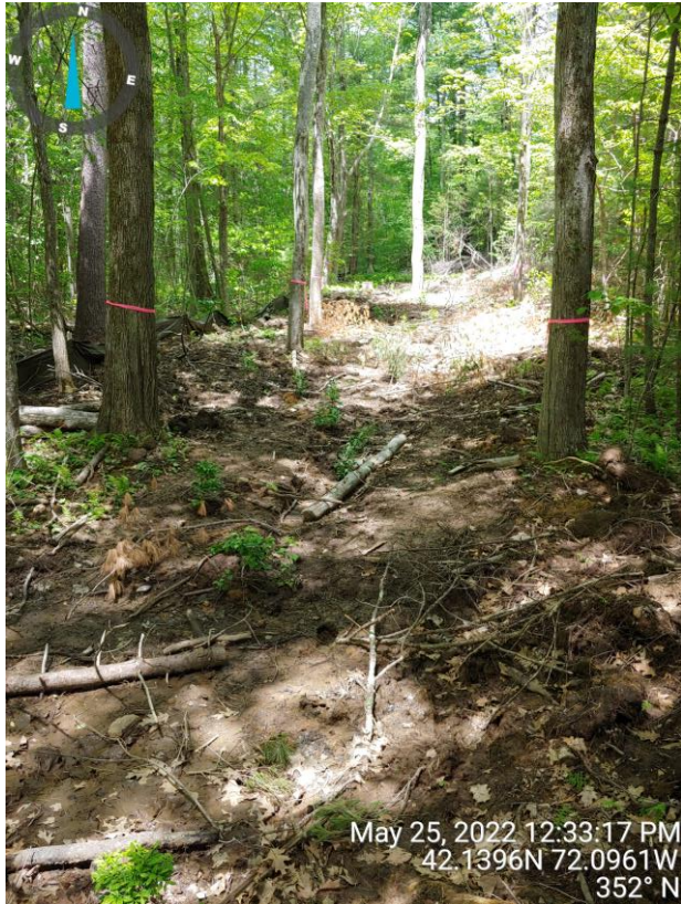
5. Finished replication area with plantings, seeding and woody material
