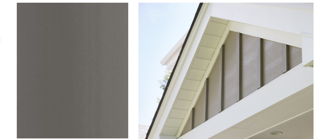
VERTICAL SIDING AT GABLE ENDS
