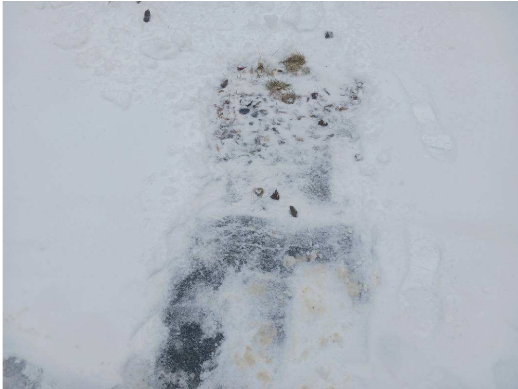
Figure 5: Cleared edge of driveway showing gravel stone diaphragm
