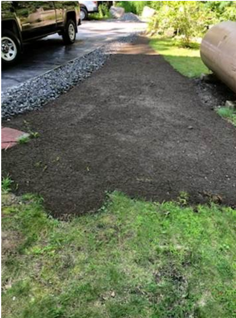
Photo 3 taken by EBT, Inc. on 9/7/2021 – Showing the 2' wide by 1' deep drip strip on the east side of the driveway.
