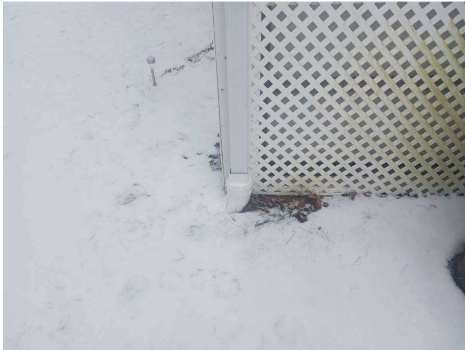
Figure 4: Roof Discharge to Cultec Drywell
