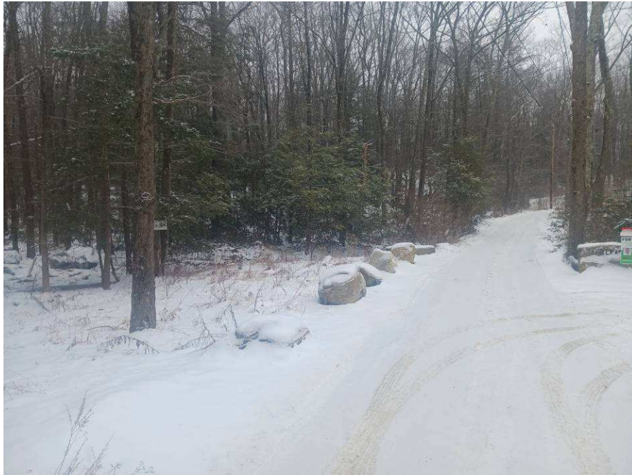
Figure 1: Boulder barrier along edge of travel way
