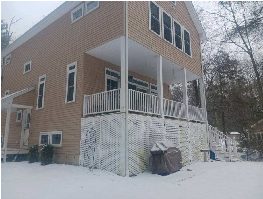
Figure 3: Roof Discharge to Cultec Drywell
