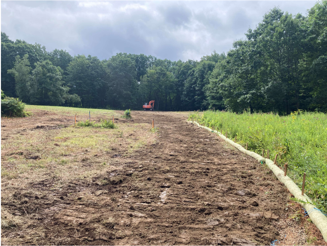
Photo 1 taken by EBT, Inc. on 8/10/2021 – Facing southeast showing the restoration area after the removal of the PVC pipe and crushed stone bed (shown on the restoration plan) was completed.
