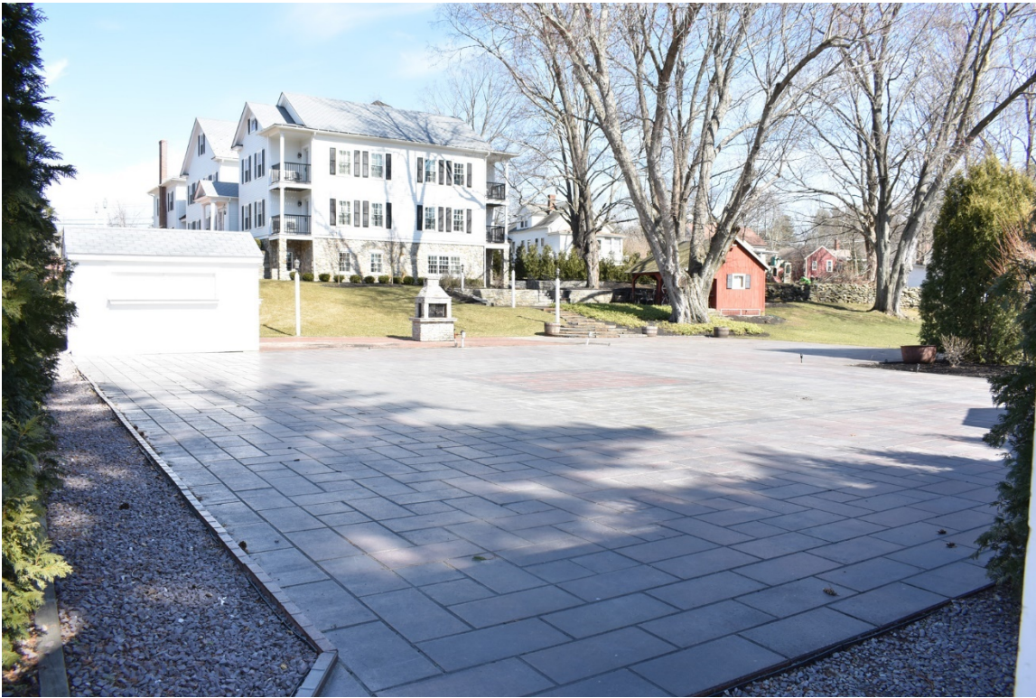
Photo 3. Stone Patio and Server Station (left), looking northeast.
