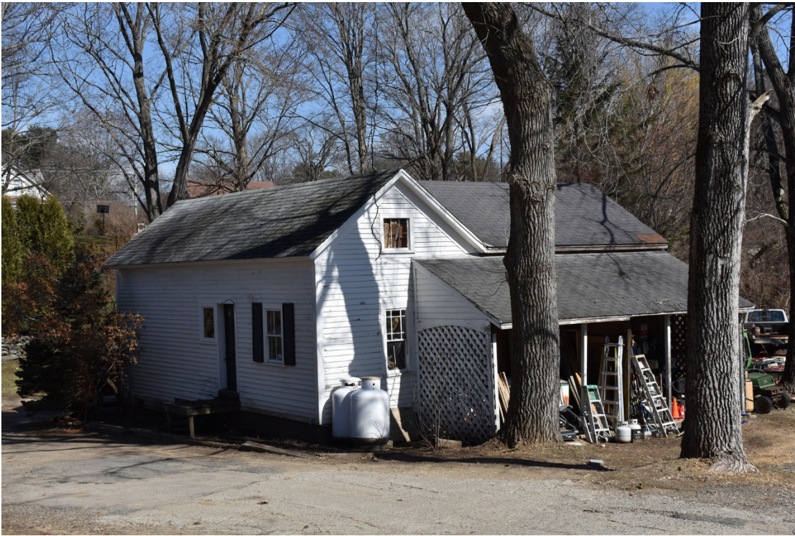
Photo 5. Maintenance Building, looking northeast.
