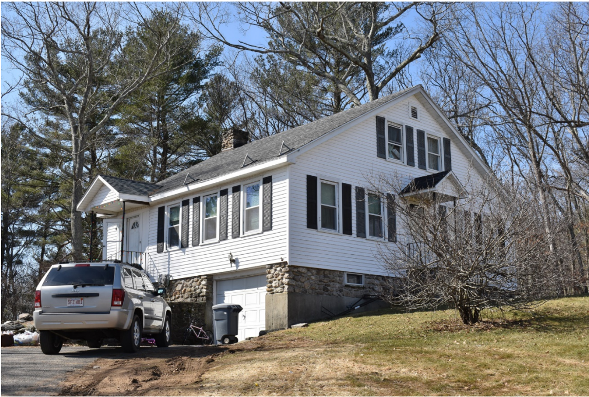
Photo 7. South Single-Family Residence, looking northwest.
