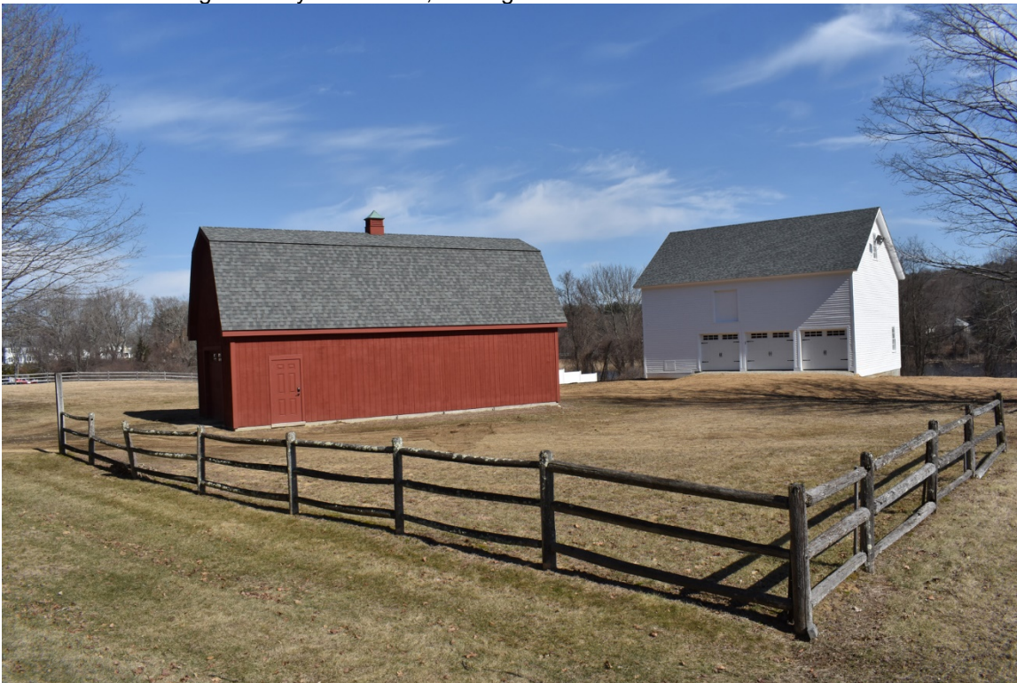
Photo 8. A. B. Chamberlain Grain and Feed Barn (right) and Barn (left), looking northeast.
