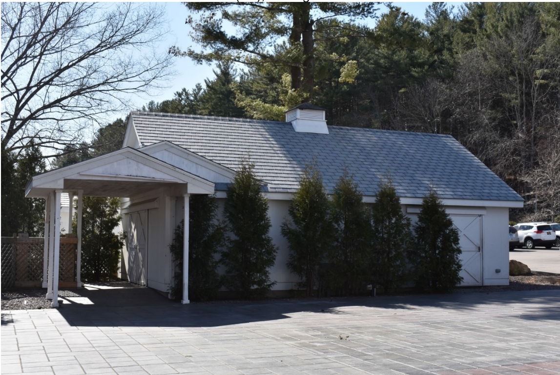
Photo 4. Prep Kitchen, looking southwest.
