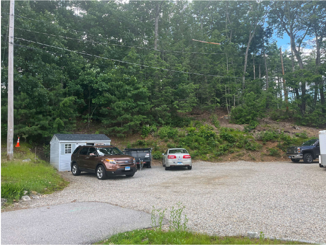
Photo 1 taken by EBT, Inc. on 6/21/2023 – Showing hill to be excavated for new garage and shed to be moved to the northwest side of the house.
