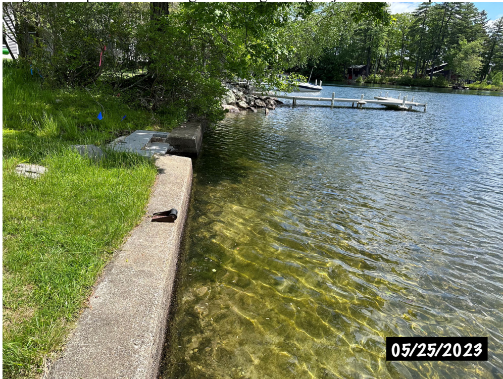
Looking northeast along the cement retaining wall towards the replication area
