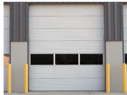
Aluminum full view sections all for maximum natural light and visibility
