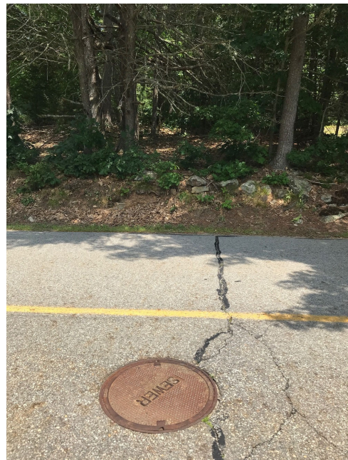
Frontage on Cedar Street / Gravity Sewer Manhole
