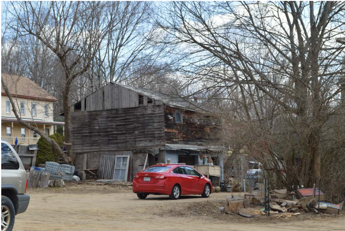
Photo 2. Garage, 552 Main Street, looking southeast.
