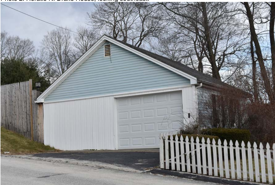
Photo 3. Garage, looking northeast.
