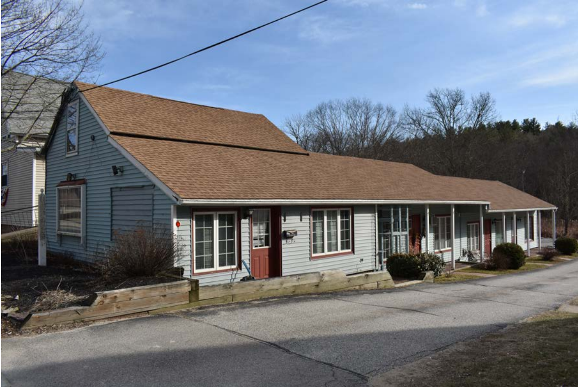
Photo 2. Hayward Barn (STU.182), 509 Main Street, looking southeast.
