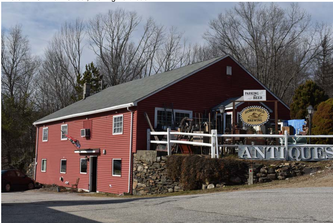
Photo 3. Barn, 484 Main Street, looking northwest.
