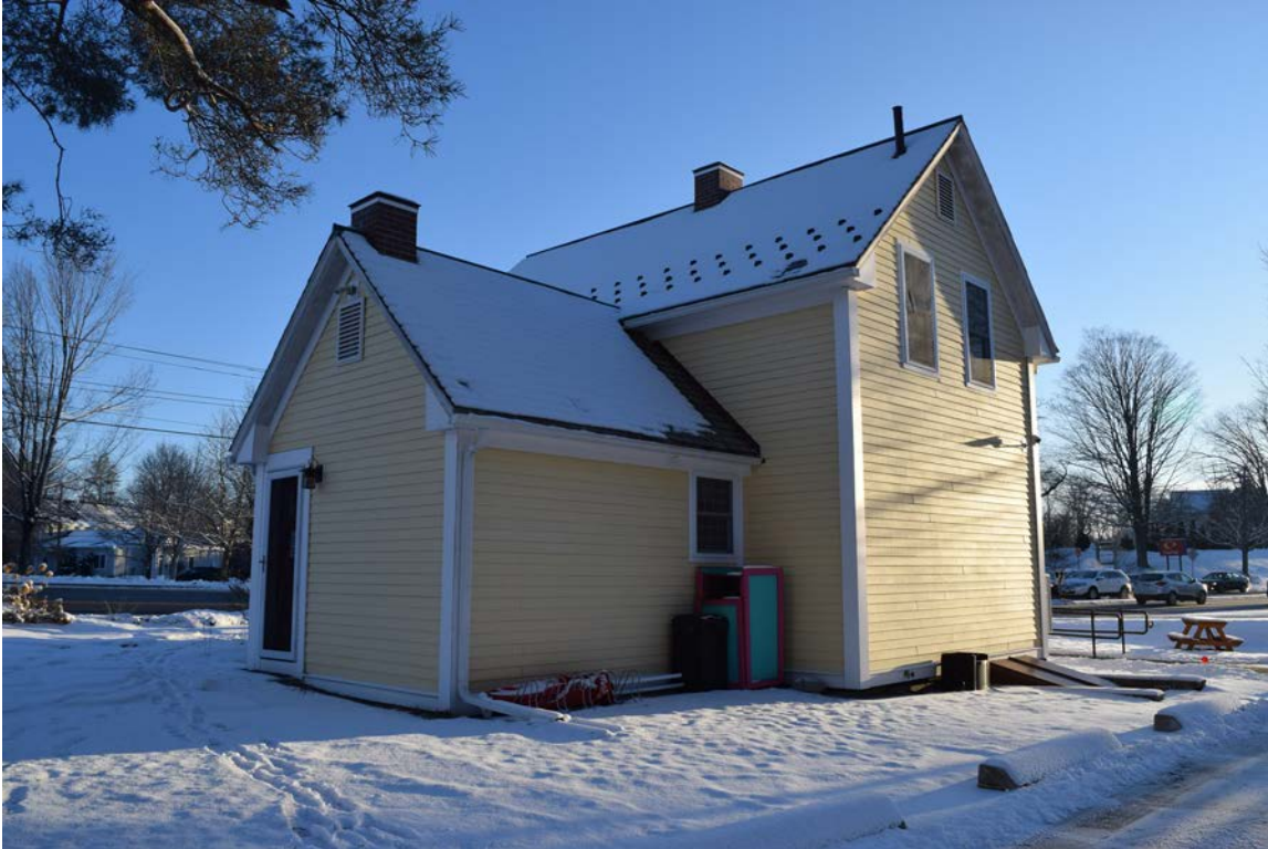
Photo 2. 413 Main Street, looking northeast.
