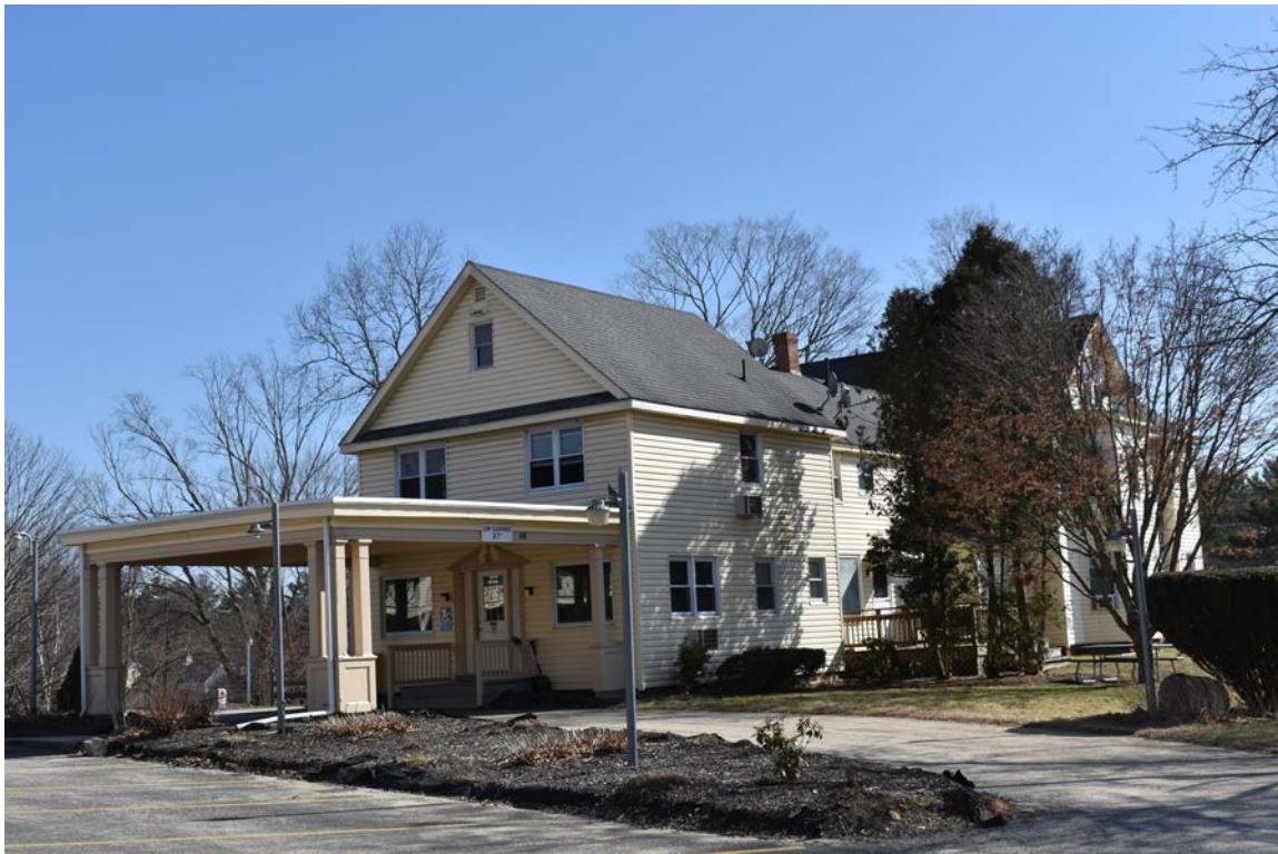
Photo 2. 408 Main Street (STU.84), looking southeast.
