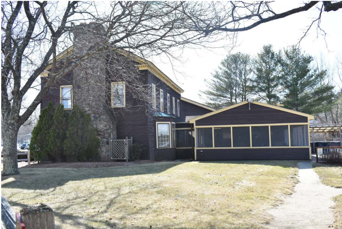
Photo 2. Brimfield Congregational Church Conference Hall, looking southwest.
