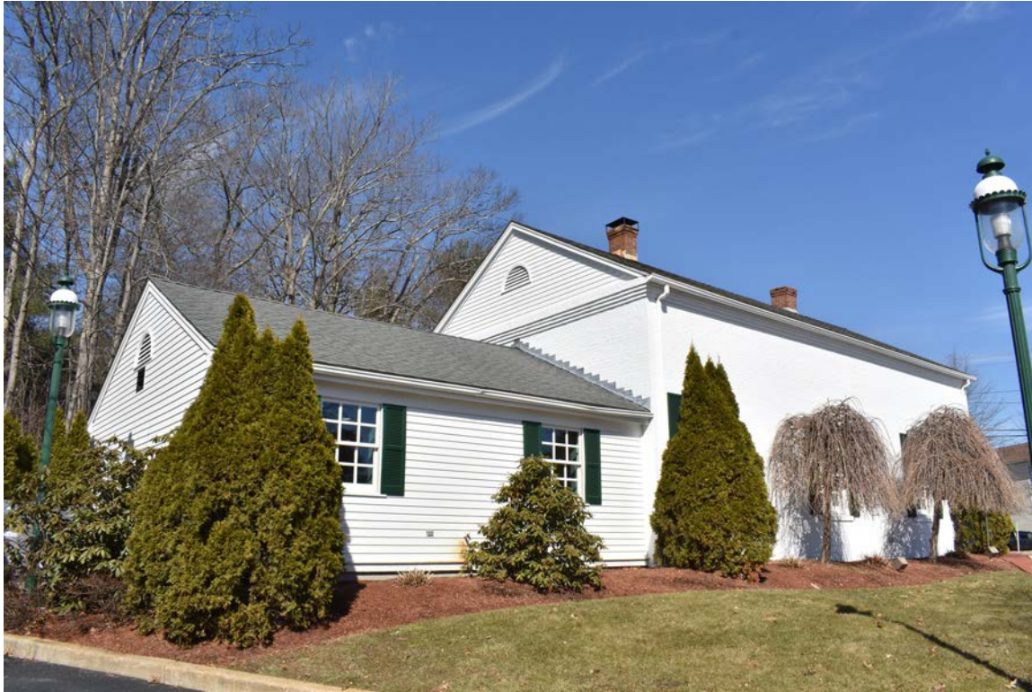
Photo 2. Southbridge and Sturbridge Street Railway Substation, looking north.
