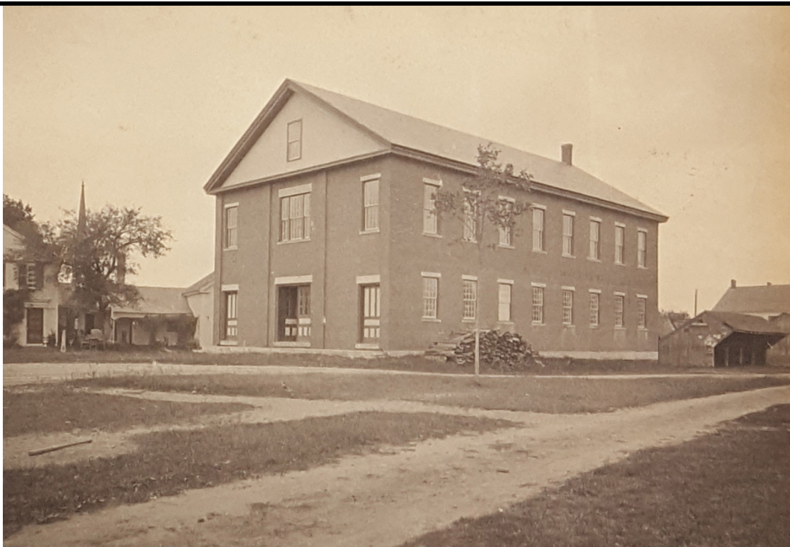
Figure 2. Sturbridge Town Hall, ca. 1900; to the left is 310 Main Street, and to the right is a small hitching shed (no longer extant) (State Library of Massachusetts).
