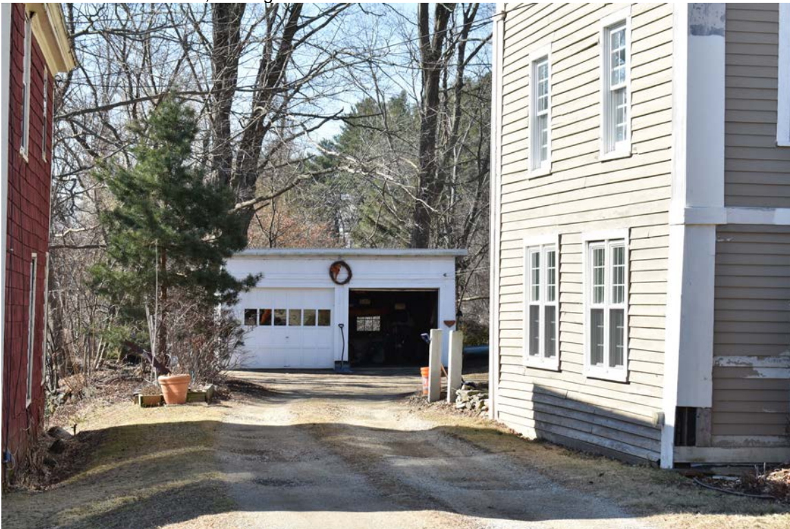
Photo 3. Garage, 269 Main Street, looking southwest.
