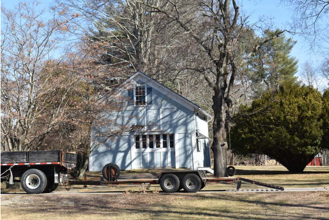
Photo 2. Barn, 266 Main Street, looking northeast.
