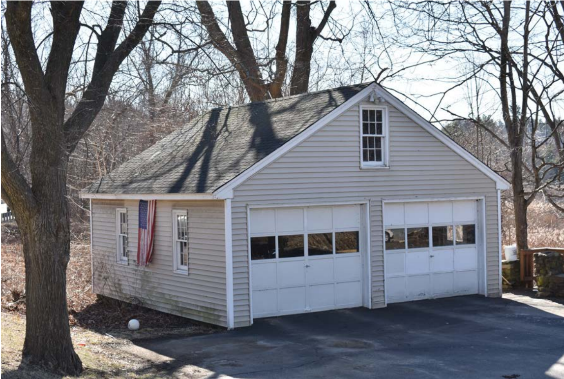
Photo 2. Garage, looking southeast.
