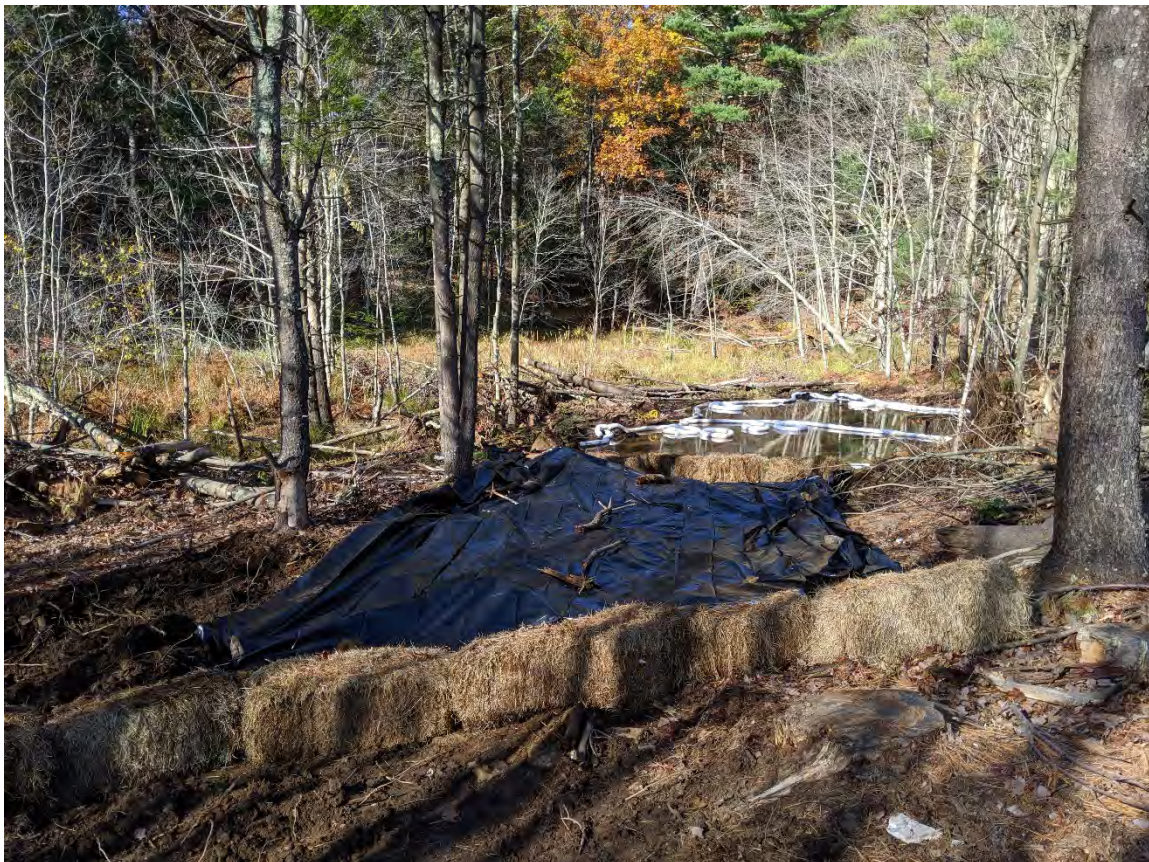
Photograph 39: View of temporary erosion controls, looking west. (10/23/2019)
