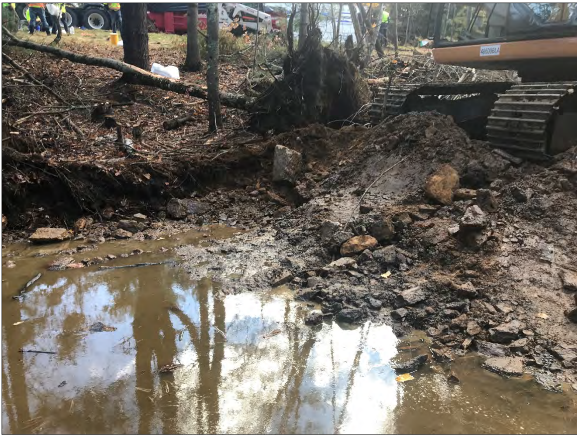
Photograph 33: Impacted soil removal activities, looking southeast. (10/23/2019)
