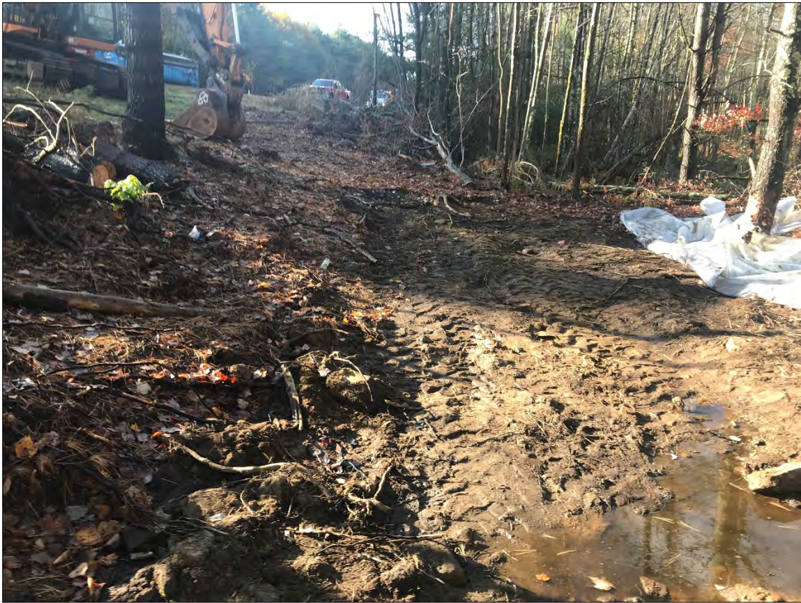
Photograph 31: Close up view of truck accident footprint, looking south. (10/23/2019)
