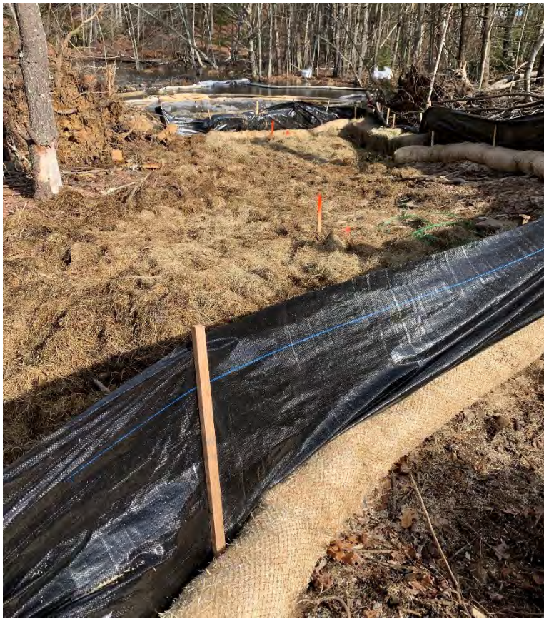
Photograph 40: View of erosion controls installed along areas of disturbance, looking west. (02/12/2020)
