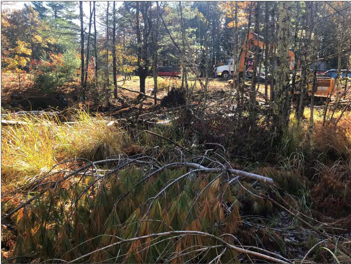
Photograph 27: View of slope down from I-84 Eastbound, looking northeast. (10/23/2019)
