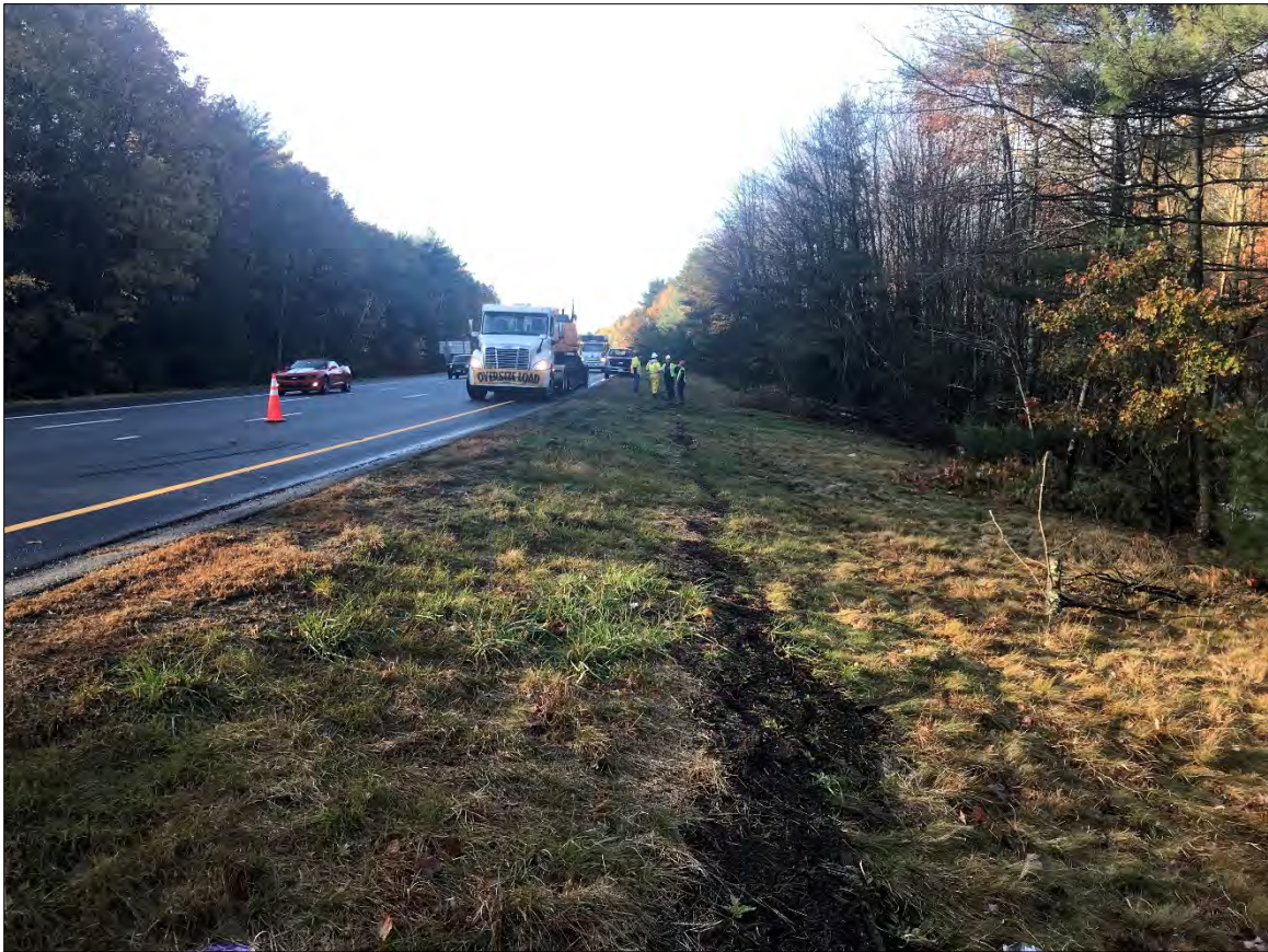
Photograph 1: View of I-84 Eastbound, looking southwest. (10/23/2019)
