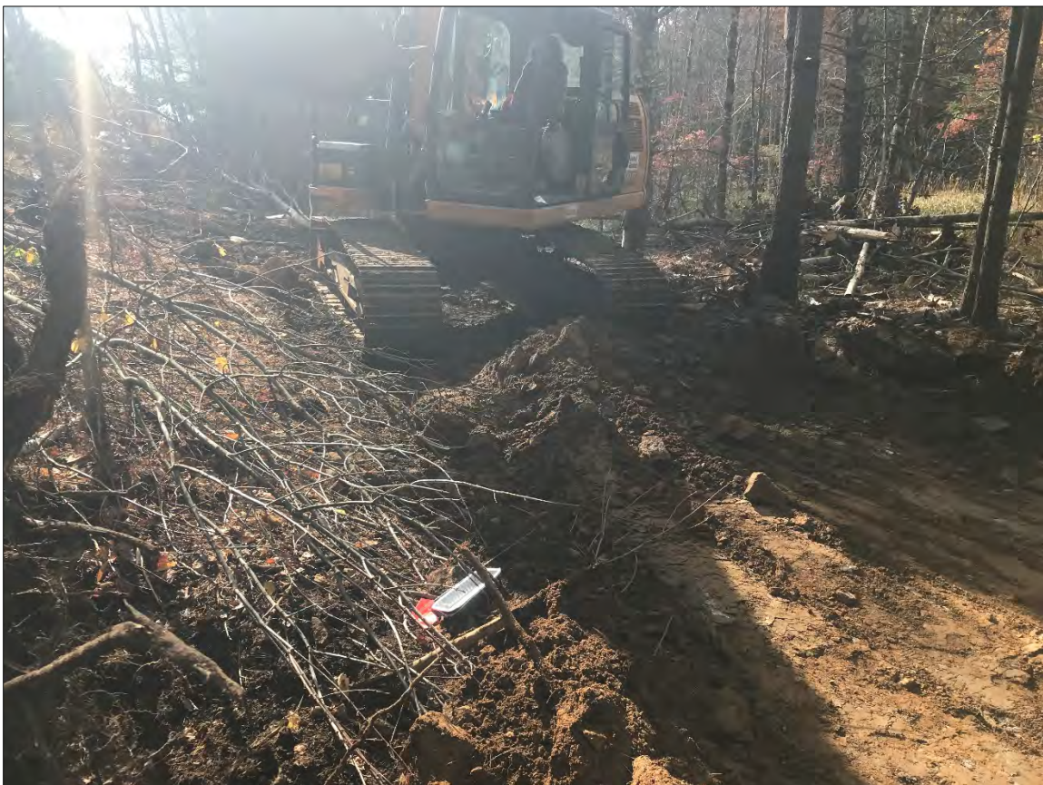
Photograph 34: Impacted soil removal activities, looking southwest. (10/23/2019)
