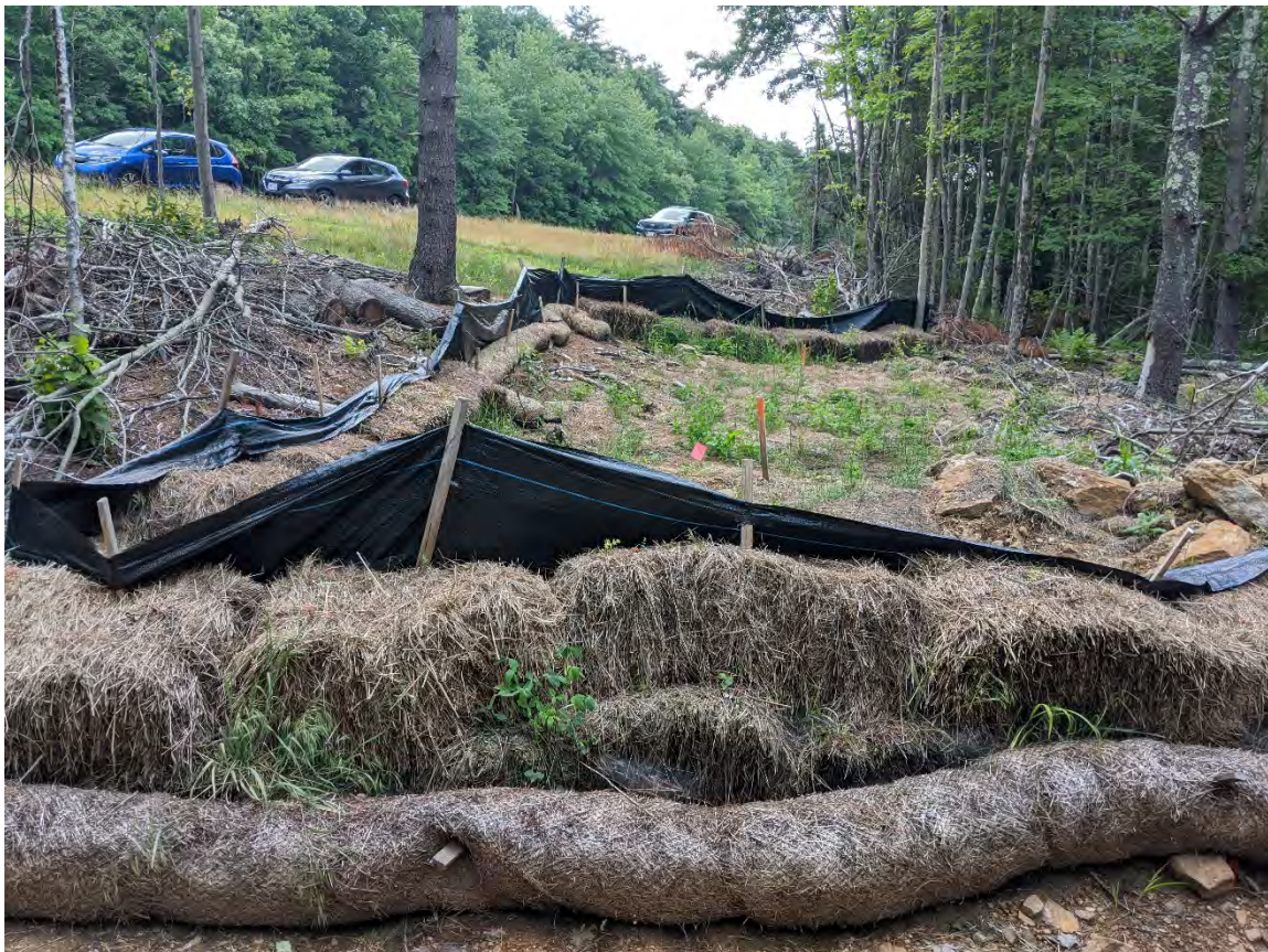
Photograph 41: View of erosion controls installed along areas of disturbance, looking east. (07/09/2020)
