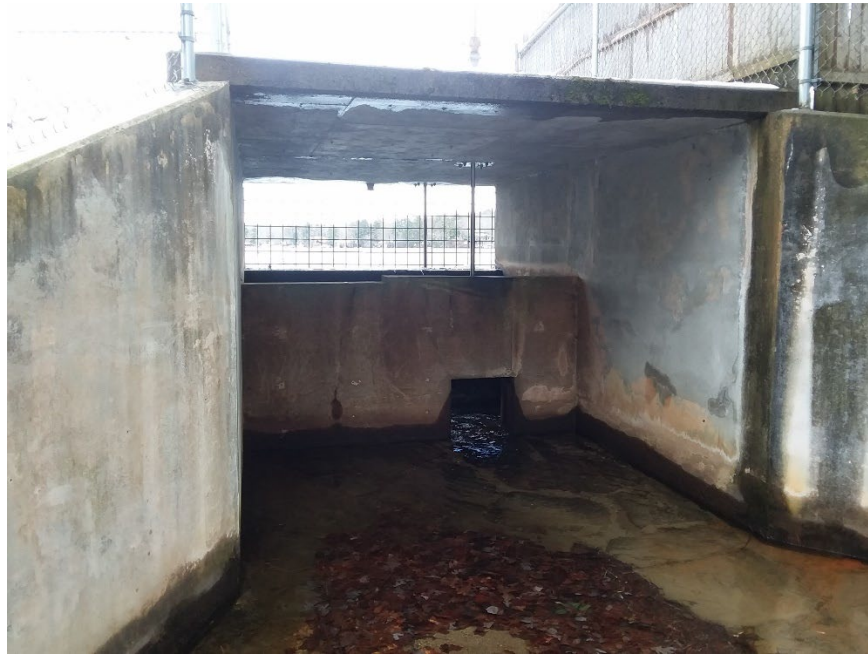
Photo 1: The 2' X 2' opening where water flows out.
