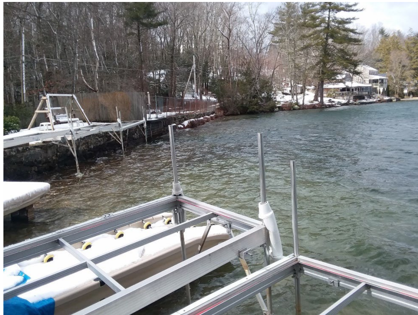
Photo 4: View of the dam, looking from the southeast.
