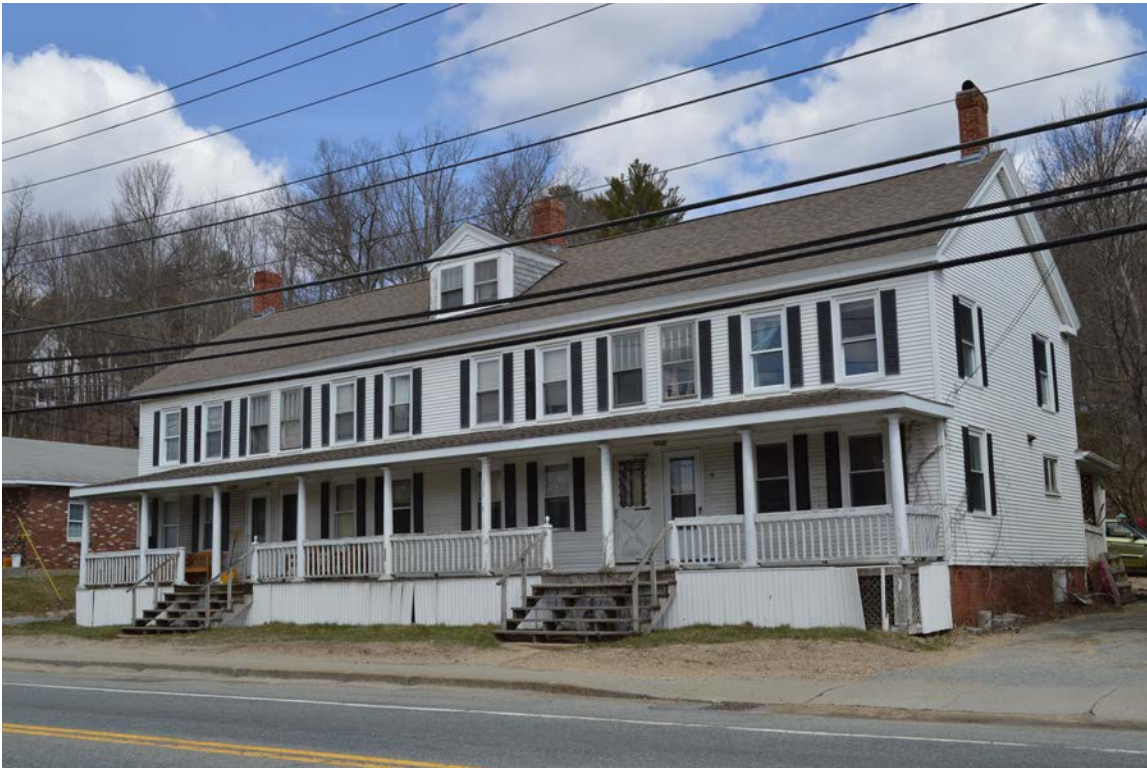
Photo 14. 554 Main Street (STU.146), looking southeast.
