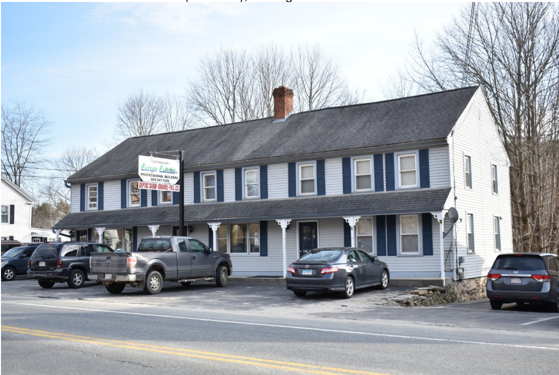
Photo 11. 537 Main Street (STU.190), looking southeast.
