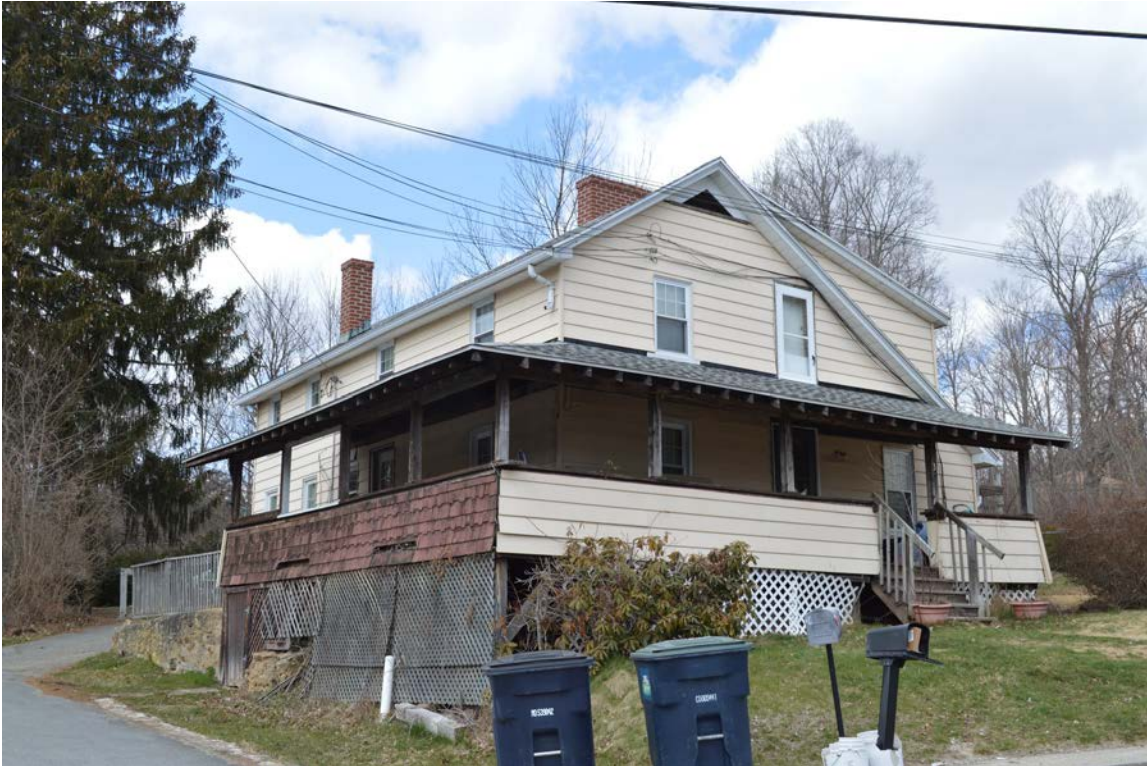
Photo 2. 3 Church Street (STU.166), looking northwest.
