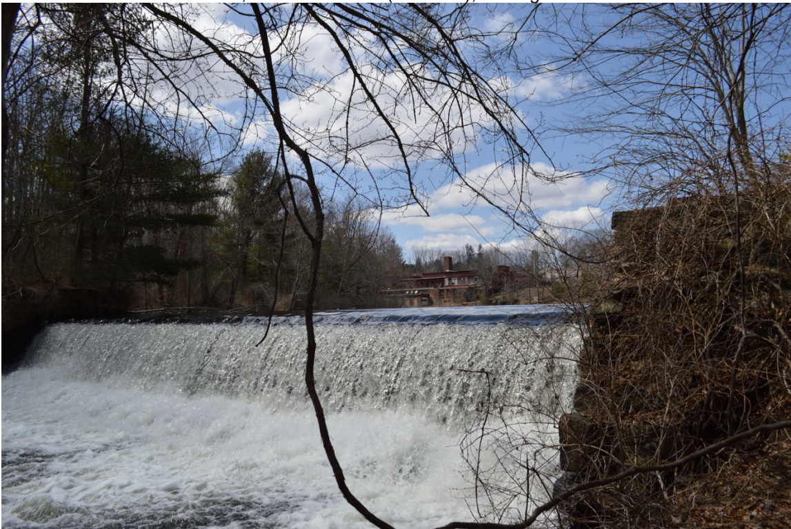
Photo 17. Sturbridge Cotton Mills Dam, South of 559 Main Street, looking southeast.
