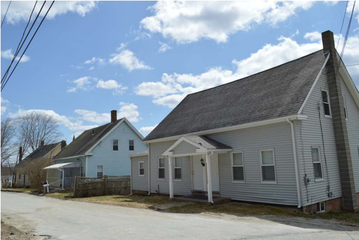
Photo 4. (R-L) 2, 4, and 6 High Street (STU.169–STU.171), looking southeast.
