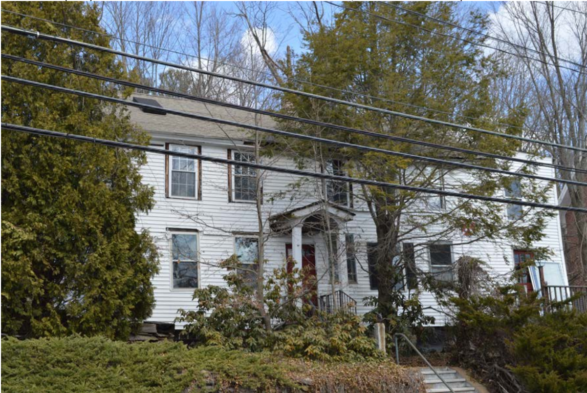
Photo 19. 584 Main Street (STU.153), looking north.
