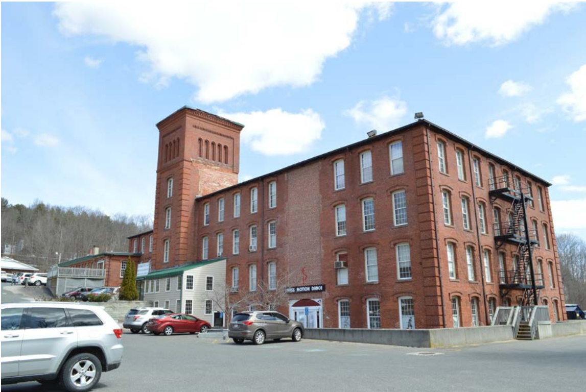
Photo 16. Fiskdale Lower Mill, 559 Main Street (STU.193), looking northeast.
