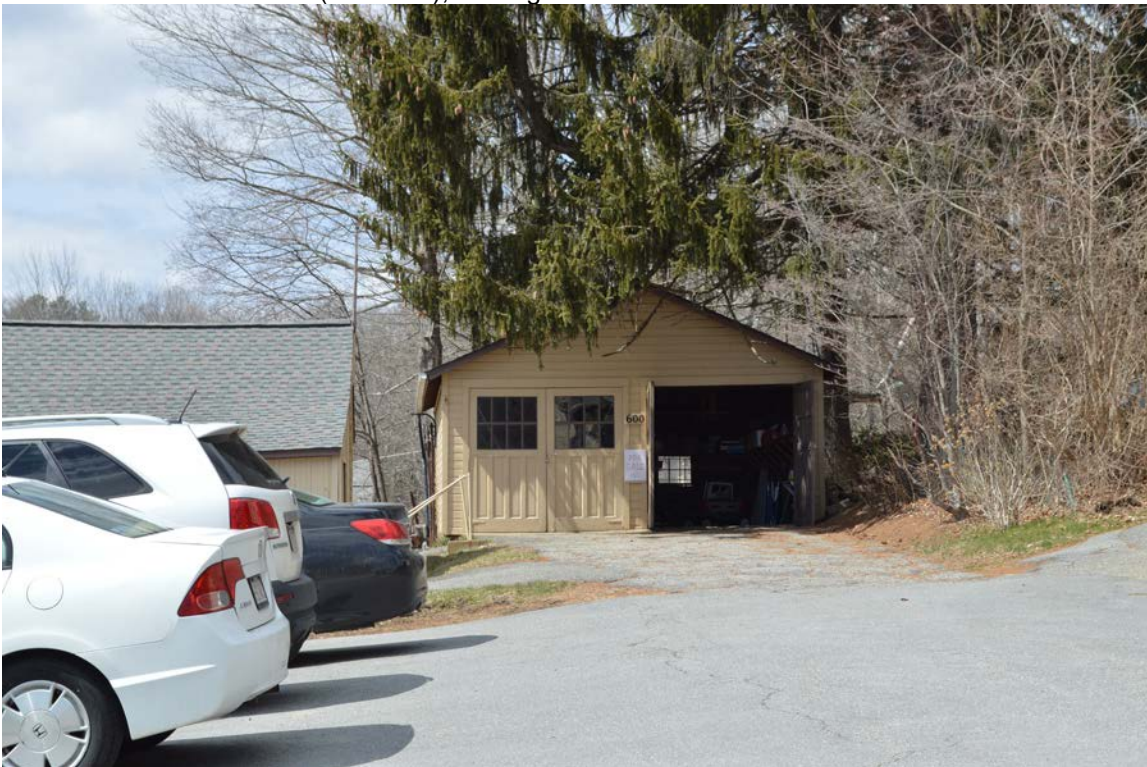
Photo 23. Garage, 600 Main Street, looking north.
