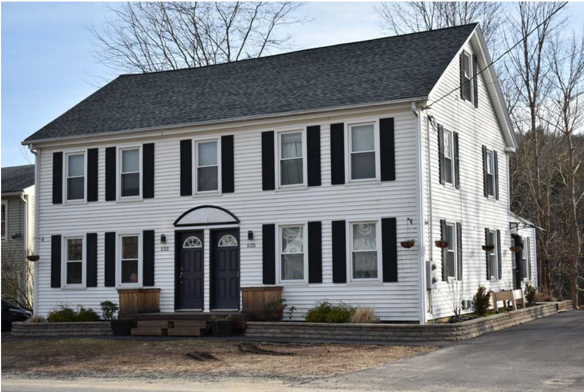
Photo 10. 533–535 Main Street (STU.189), looking southeast.
