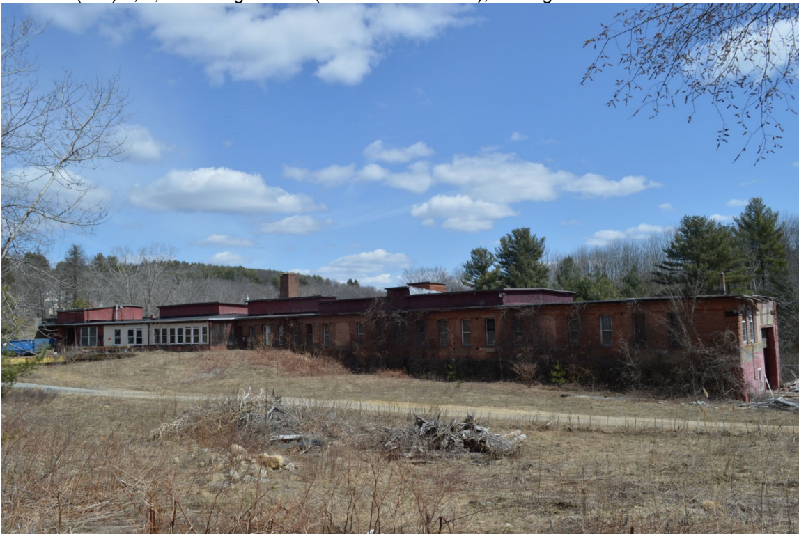
Photo 5. Fiskdale Upper Mill, 9 Holland Road (STU.194), looking northeast.
