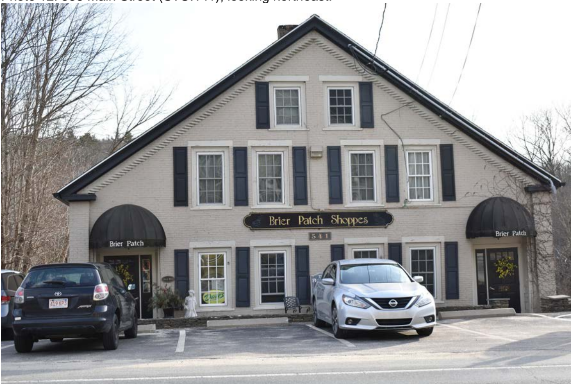
Photo 13. 541 Main Street (STU.191), looking southwest.
