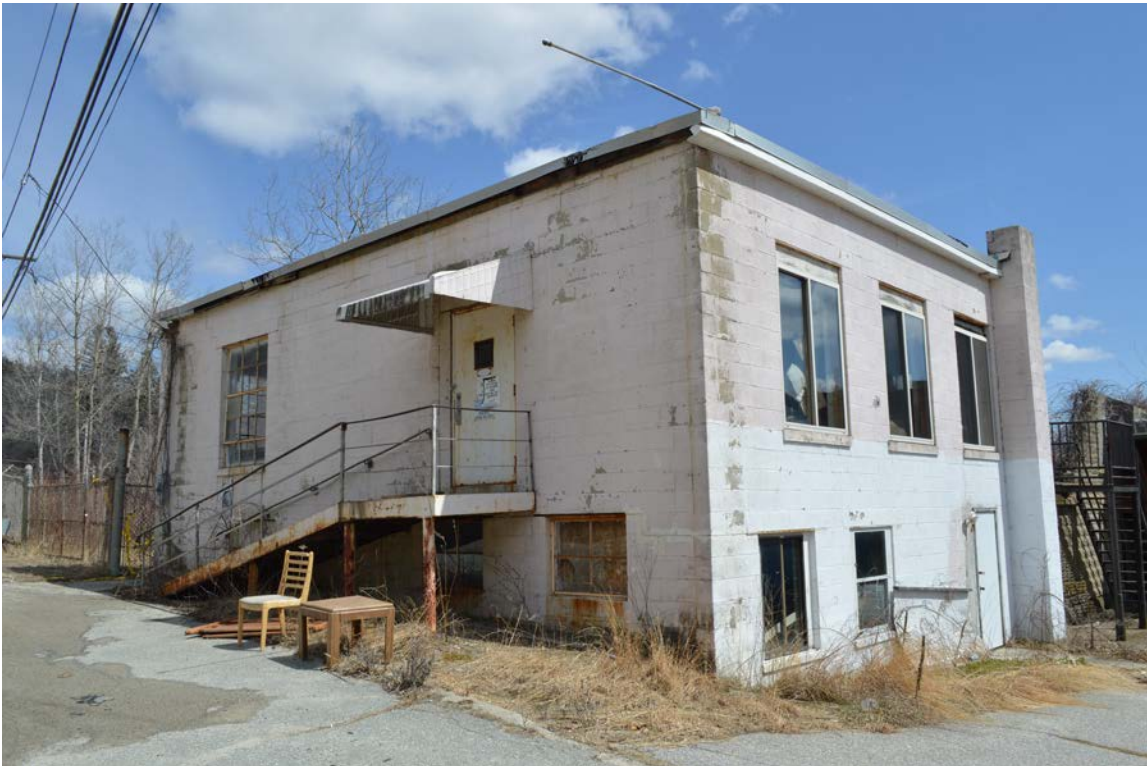
Photo 6. Post-1933 concrete-block addition to Fiskdale Upper Mill, 9 Holland Road (STU.194), now separated from the mill by demolition of Mill No. 1 and Mill No. 1-O (see Figure 3), looking northeast.
