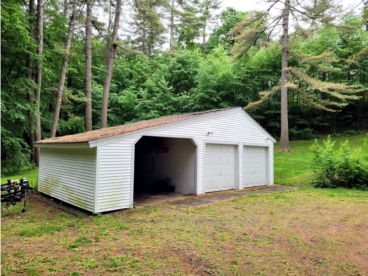
Existing Garage – 168 Lane Seven
