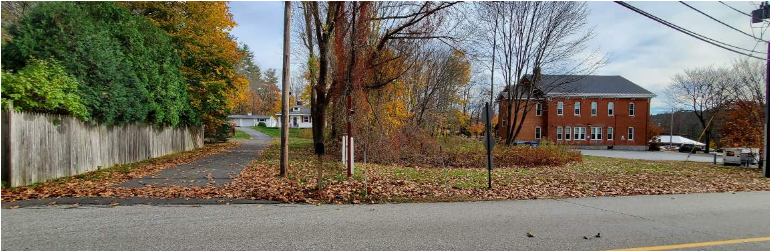
SENIOR CENTER SEEN FROM ARNOLD ROAD WITH ABUTTING NEIGHBOR
