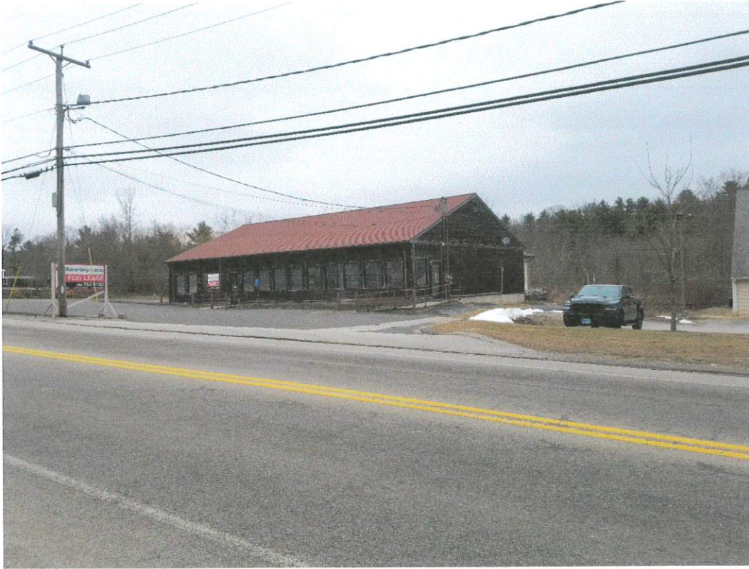
WEST & SOUTH BUILDING ELEVATIONS & FRONT PARKING AREA (Looking Northeast Toward Property)
