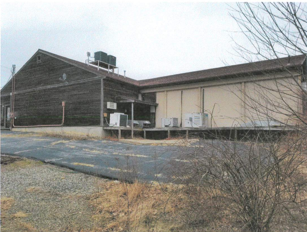
SOUTH BUILDING ELEVATION (Looking Northwest Toward Property)
