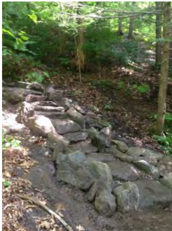
Stone staircase installed by SCA at Mohawk state forest
