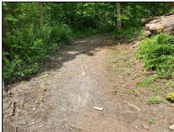
Photo 8. View facing west showing an area of erosion in the trail. This is proposed to be spot-graded to reduce cross slope and protect downgradient resource areas. Photograph taken May 26, 2022.
