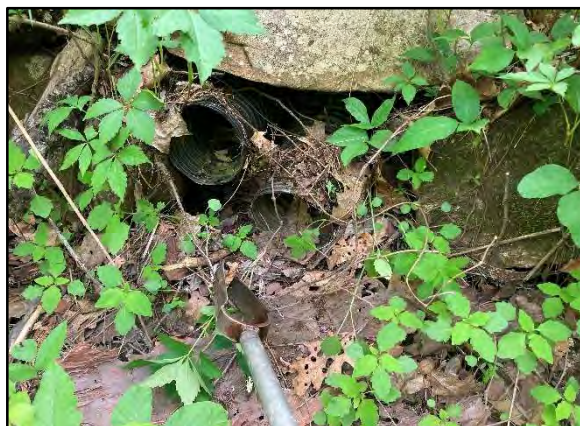
Photo 6. Overflow plastic culverts at Stream S3 crossing. Photograph taken May 26, 2022.
