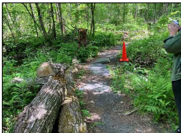
Photo 4. View facing northeast at the trail crossing with Stream S3. DCR proposes to add a wooden puncheon here this. Photograph taken May 26, 2022.
