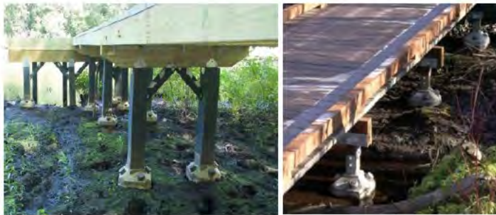
Photo #6: View of an example of a diamond pier wooden puncheon installed in a wetland.
