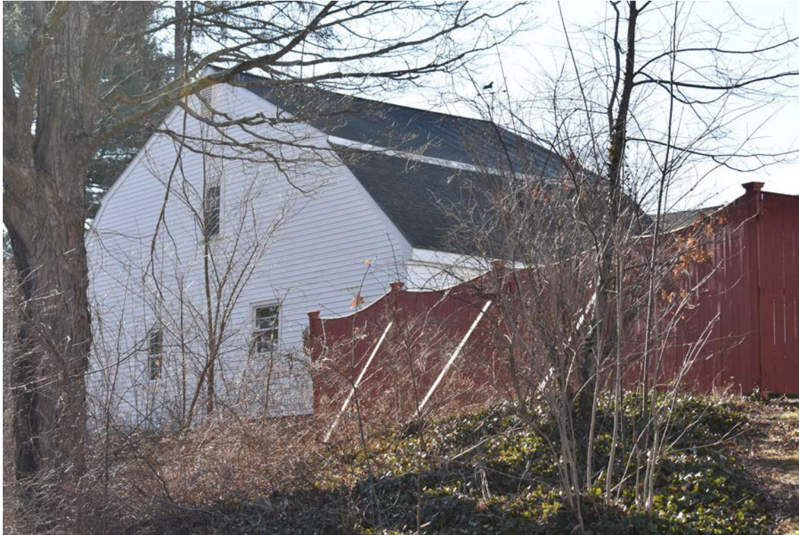
Photo 2. George Davis Barn, 10 Charlton Street, looking southeast.
