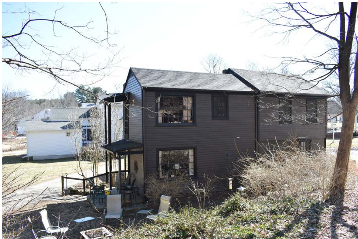
Photo 2. 12 Chamberlain Avenue, looking southeast.
