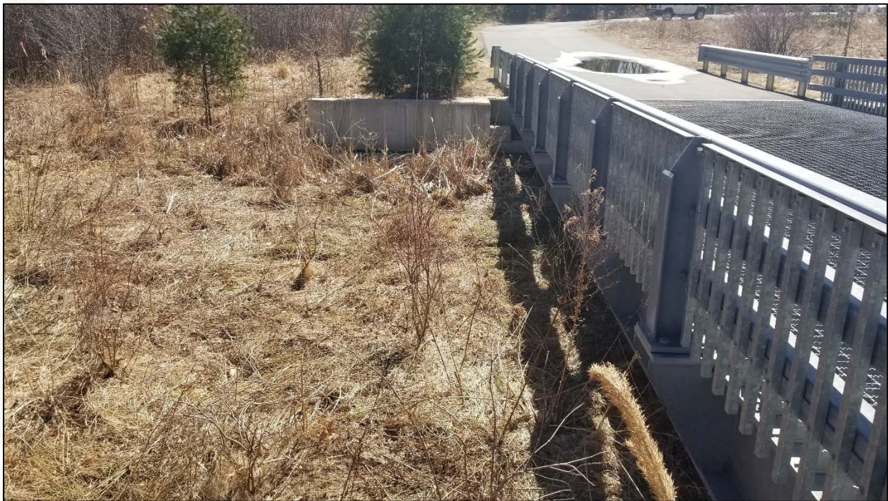
Photo 1: Grated bridge spanning BVW between two vernal pools supporting rare amphibians. Source: Oxbow Associates, Inc.
