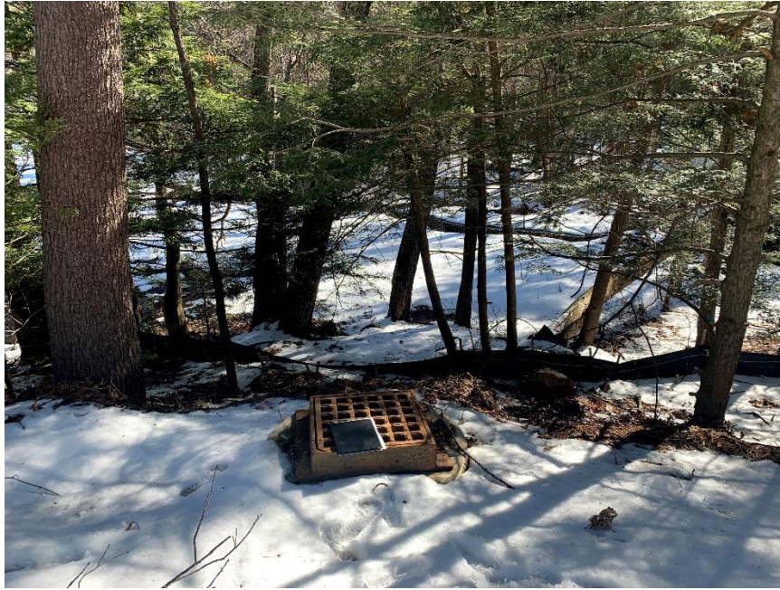
Figure 1: Looking at Hydrodynamic Separator East Toward Pond
