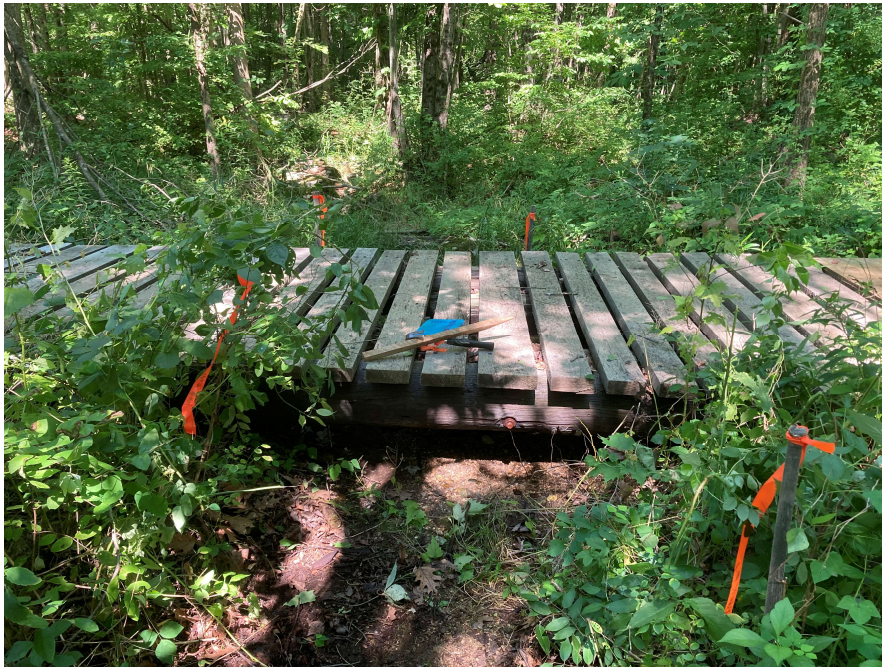
Photo 2 taken by EBT, Inc. on 7/19/2020 – Showing the general spacing of the 2” planking and the 8” height of the bottom of the pole at the brook flow location over the intermittent stream bottom.
