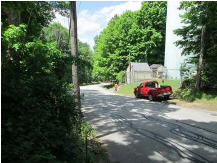
Fiske Hill Water Booster Station (Photo No. 3576)
