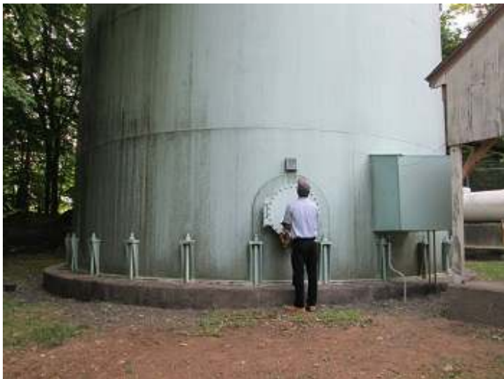
391,000 Gallon Storage Tank (Photo No. 4438)
