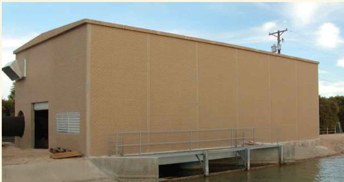
Unobstructed 30' W x 24' H x 60' L space allows room for large hydroturbine equipment, Mesa, AZ
