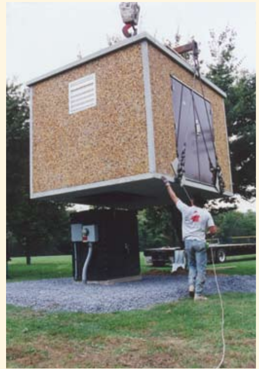
Transformer Substation (Pre-assembled building delivered with hole in floor to fit over transformer)
