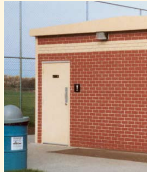
Combination concessions and restrooms
