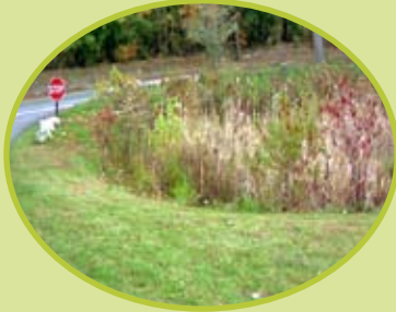
Constructed Stormwater Wetlands
