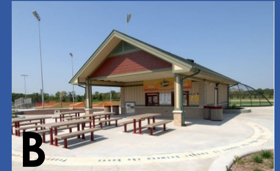
B FIELD SUPPORT BUILDING
