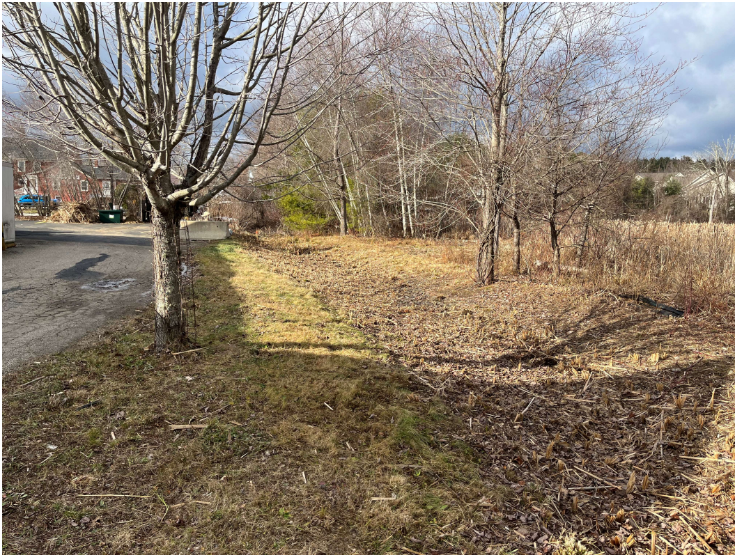
Photo 1 taken by EBT, Inc. on 12/19/2022 – Water quality swale behind the building running in an east to west direction. The swale has been cleared of herbaceous vegetation & trash and mowed. Once we receive the existing conditions plan from Levesque Geomatic, we will understand if the swale meets the original design from Andrews Surveying and Engineering's revised 2005 plan.
