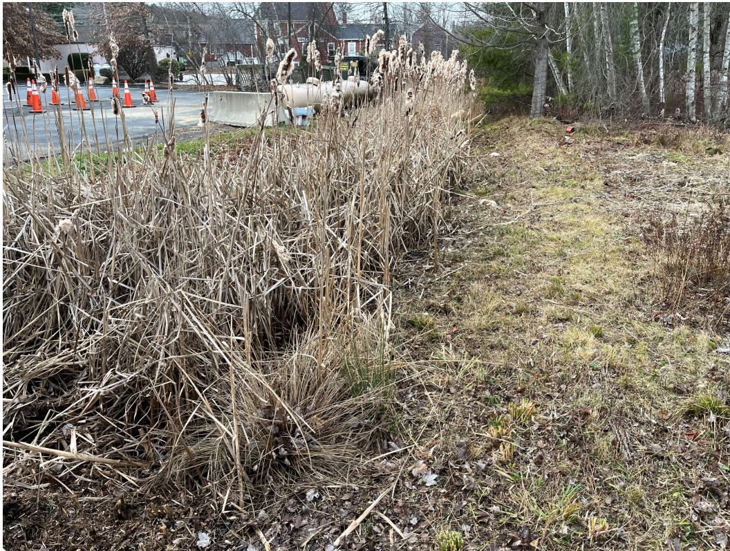
Photo 3 taken by EBT, Inc. on 12/4/2022 – Portion of water quality swale prior to clearing and mowing.
