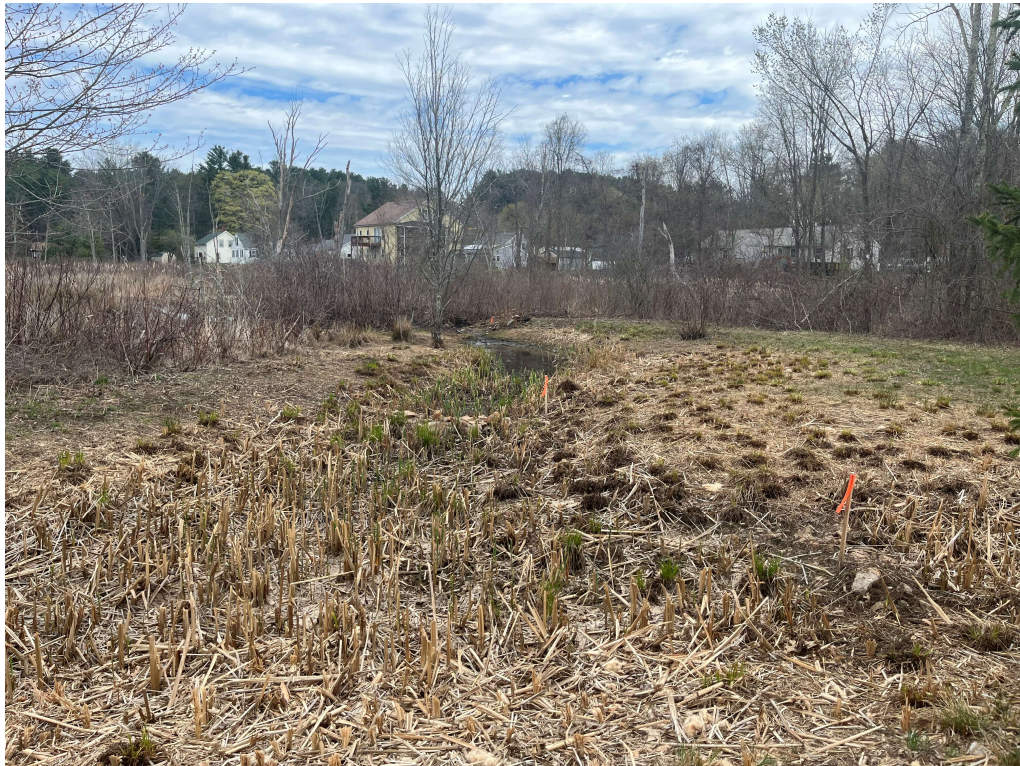
Photo 1 taken by EBT, Inc. on 12/19/2022 – Water quality swale behind the building running in an east to west direction. The swale has been cleared of herbaceous vegetation & trash and mowed. Once we receive the existing conditions plan from Levesque Geomatic, we will understand if the swale meets the original design from Andrews Surveying and Engineering's revised 2005 plan.
