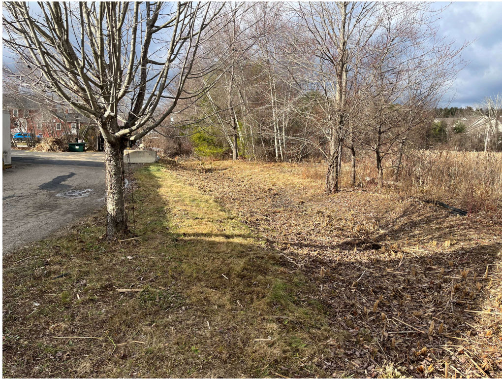
Photo 1 taken by EBT, Inc. on 12/19/2022 – Water quality swale behind the building running in an east to west direction. The swale has been cleared of herbaceous vegetation & trash and mowed. Once we receive the existing conditions plan from Levesque Geomatic, we will understand if the swale meets the original design from Andrews Surveying and Engineering's revised 2005 plan.
