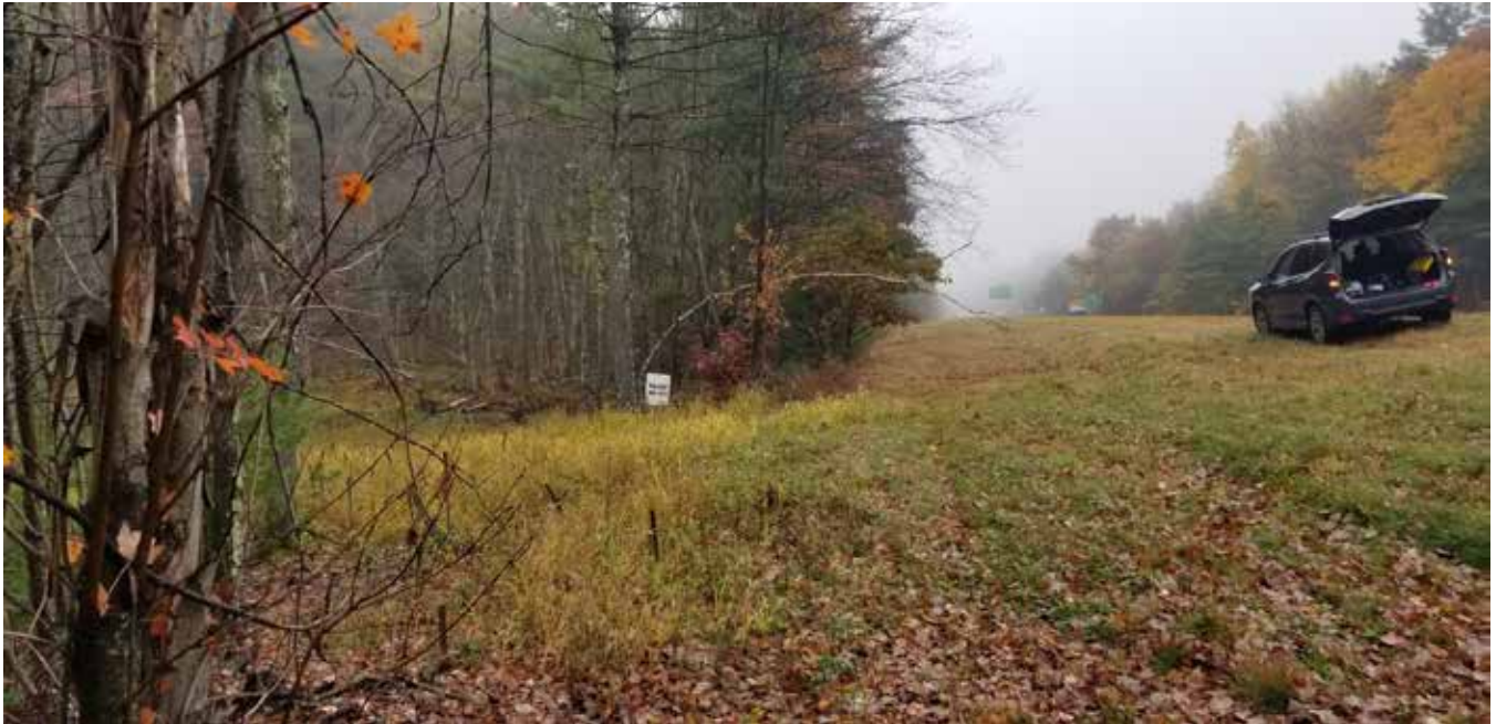
Photograph 1: View of I-84 Eastbound and erosion control mats on edge of highway, looking northeast.
