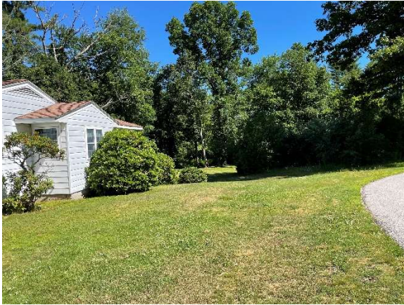
Description: Site North Facing 1
