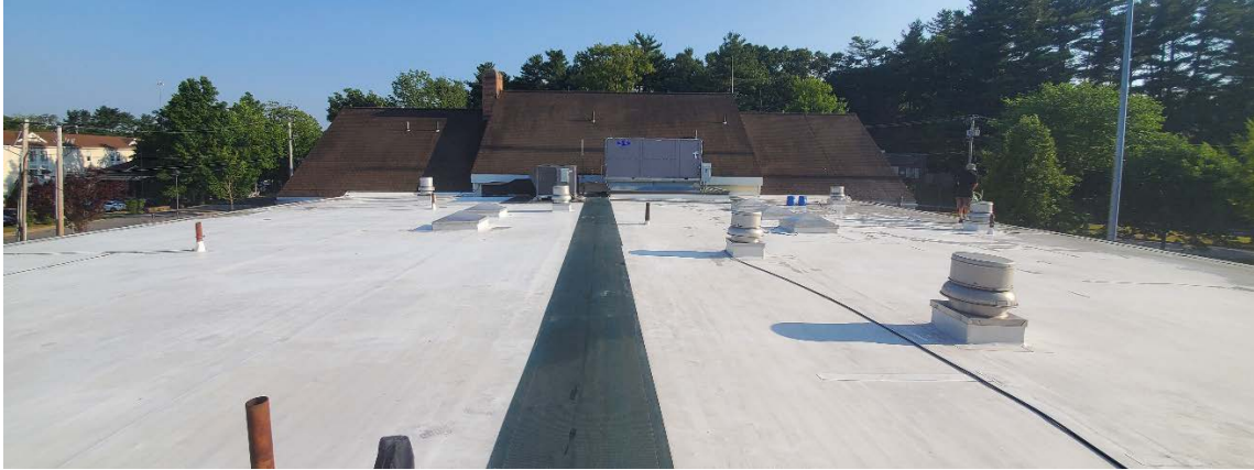
Public Safety Roof after powerwashing
