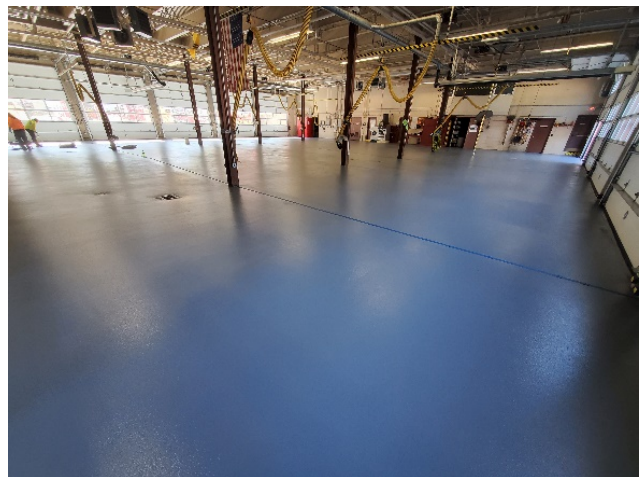
Apparatus Floor After
