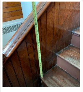
Guardrail at second floor has been amended in height but may not meet code lateral force requirement. It's opening exceeds the 4" sphere requirement and does not have a compliant rail shape.
