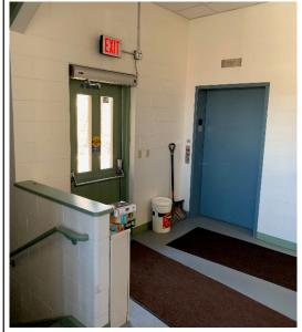
Exterior door from office at southeast corner is equipped with a panic bar but is not identified as an exit.
