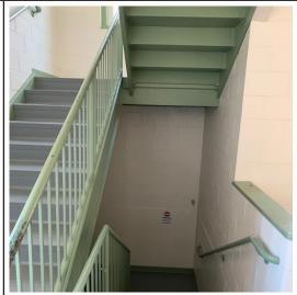
The basement corridor leading to the north stair is 34" in width. 2015 IBC Table 1020.2 requires a minimum corridor width of 36" for an occupant load less than 50 people. The fintube radiant heat register further restricts the corridor width.
