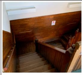
Handrail is 24" above tread nosing; it should be 2'-10". Handrail shape is non-compliant.
