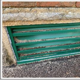
Gaps between joints in the granite foundation require re-pointing. There is a significant amount of staining on the foundation and brick at the stair addition. Observation of the roof was limited but noted that snow guards are present but there are no gutters or downspouts.
