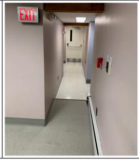
The door to the north egress stair is set deeply in excess of 6" into the original masonry foundation wall and does not comply with MAAB 26.6.2 and does not provide 12" minimum on the push side as required by 26.6.3 Fig. 26e. This door is not compliant as an accessible door to the elevator beyond.
