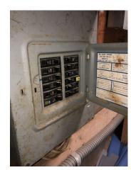
Photo 18 - Basement Load Center with Rust
