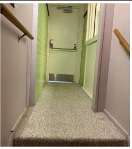
The second stair to the basement is non-compliant for width (stair narrows at top), and headroom. Handrails do not extend beyond the top and bottom riser as required by CMR 780 1014.6
