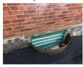
Photo 9 - Combustion Air Louver
