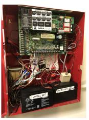
Photo 24 – Fire Alarm Panel (Exterior)
