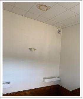
Generally, spaces on the second floor appear to be in good repair. Observations made did not identify significant physical deficiencies except for ceiling damage due to water. The Owner representative advised that paint is failing in this area.
