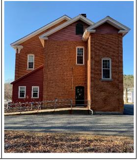
The railing at the base of the handicap ramp appears to have been hit and repaired on several occasions. The railing was in the process of being painted yellow during our site visit. There are no bollards to protect the ramp railing. The elevation difference between the asphalt pavement and the concrete ramp exceeds 1/2".
