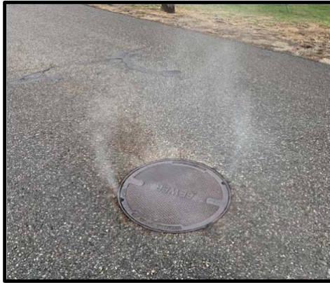
7. Hall Road - Manhole ID 215 - Vented manhole cover
