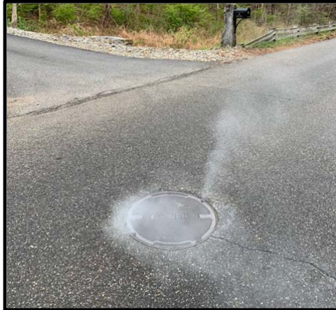
17. Hall Road - Manhole ID 226 - Vented manhole cover
