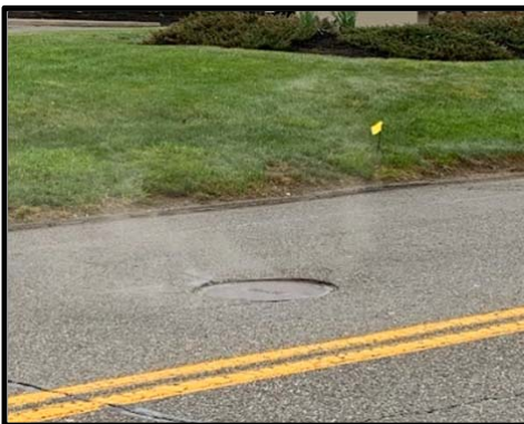
9. Hall Road - Manhole ID 217 - Vented manhole cover
