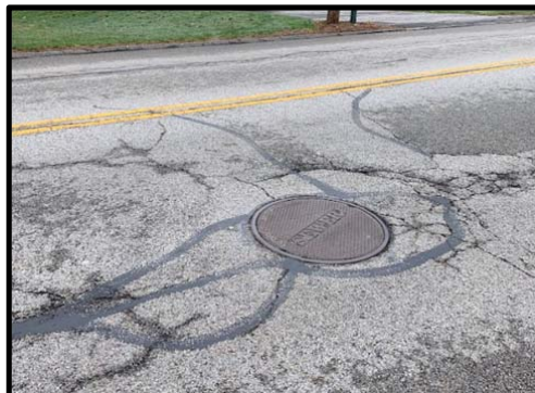
25. Whittemore Road - Manhole ID 116 - Vented manhole cover
