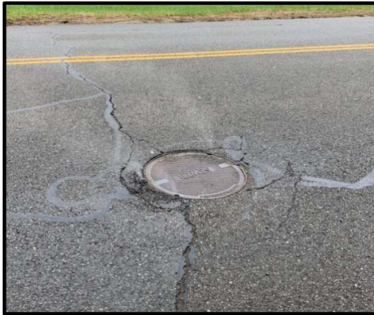
14. Hall Road - Manhole ID 222 - Vented manhole cover
