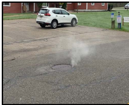
12. Hall Road Manhole ID 219 - Vented manhole cover
