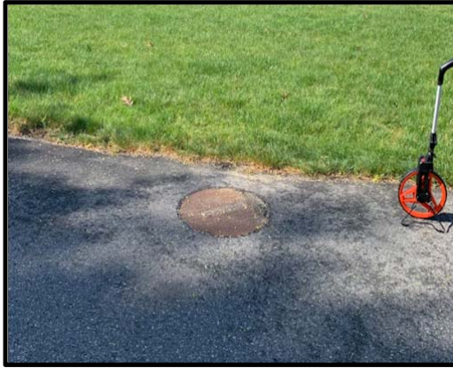
23. Old Farm Road - Manhole ID 1120 - Vented manhole cover
