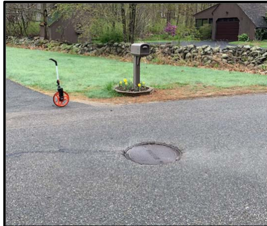
15. Hall Road - Manhole ID 223 - Vented manhole cover
