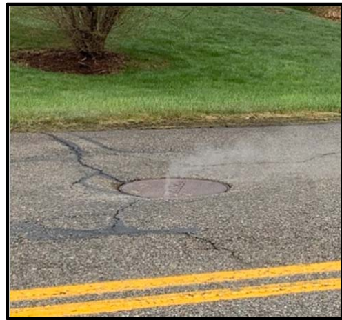
11. Hall Road - Manhole ID 218 - Vented manhole cover
