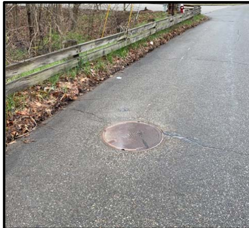
18. Hall Road - Manhole ID 227 - Vented manhole cover
