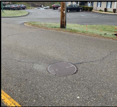
8. Hall Road - Manhole ID 216 - Vented manhole cover
