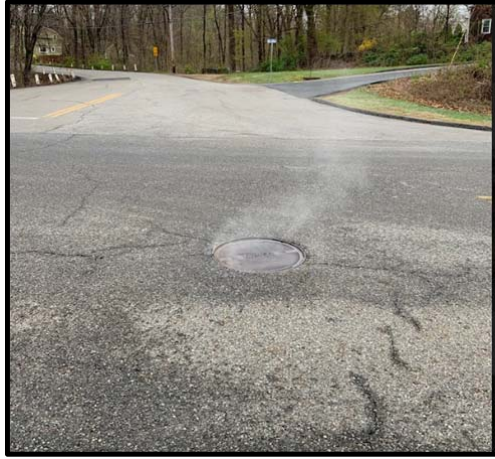
19. Hall Road - Manhole ID 120 - Vented manhole cover
