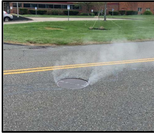
10. Hall Road - Manhole ID 597 - Vented manhole cover
