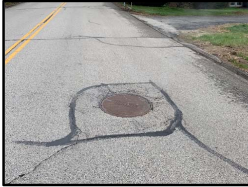
26. Whittemore Road - Manhole ID 114 - Vented manhole cover
