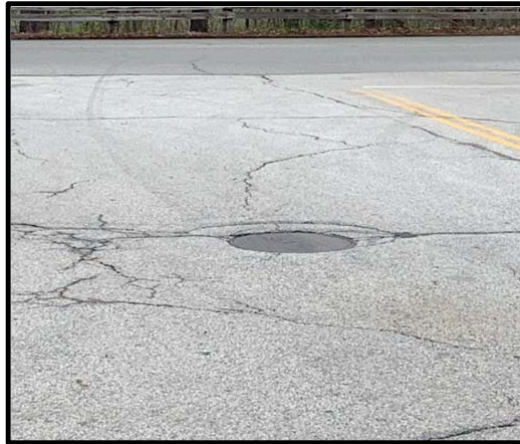
27. Whittemore Road - Manhole ID 138 - Vented manhole cover
