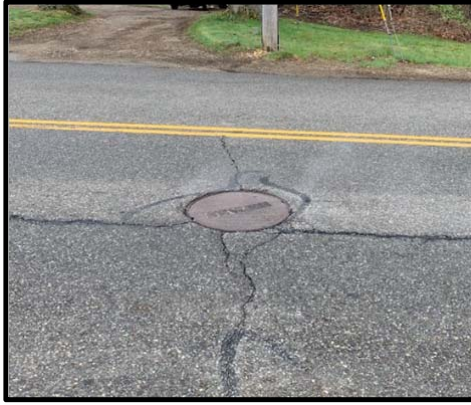
6. Hall Road - Manhole ID 1026 - Vented manhole cover
