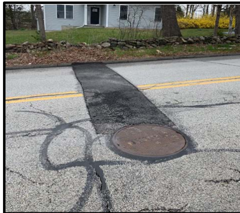
28. Whittemore Road - Manhole ID 108 - Vented manhole cover
