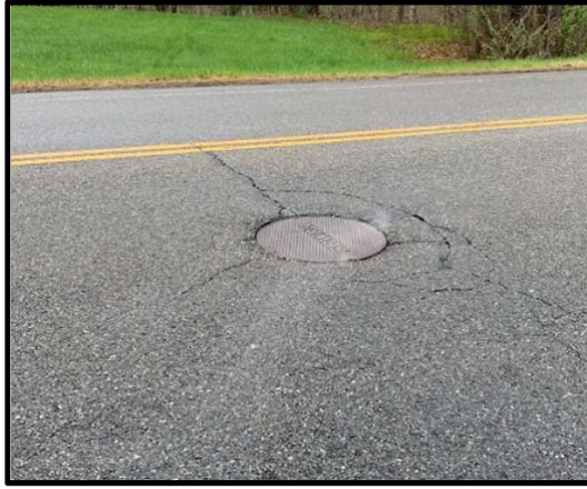
13. Hall Road - Manhole ID 221 - Vented manhole cover
