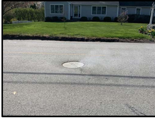
22. Old Farm Road - Manhole ID 598 - Vented manhole cover
