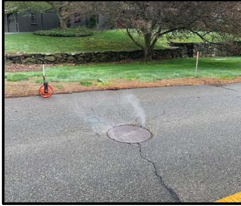
16. Hall Road - Manhole ID 225 - Vented manhole cover
