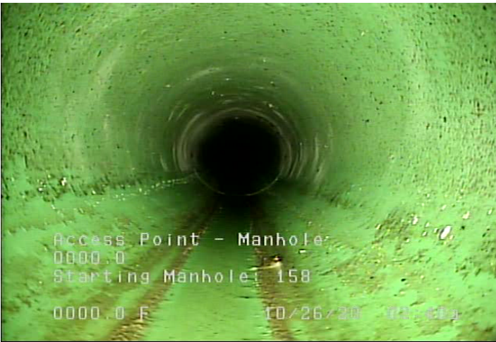
AMH - Access Point - Manhole @ 0.0 ft. Starting Manhole: 158
