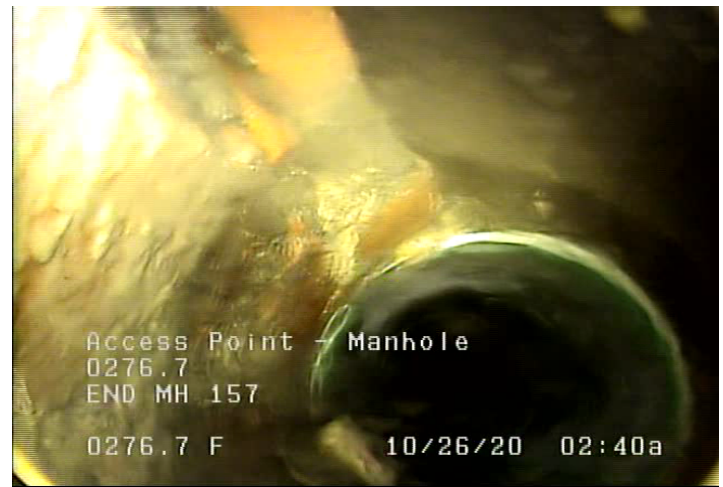
AMH - Access Point - Manhole @ 276.7 ft. END MH 157
