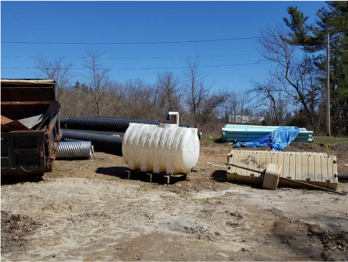
Figure 9: The area south of the Salt Shed is used for storage of drainage structures and conduit.
