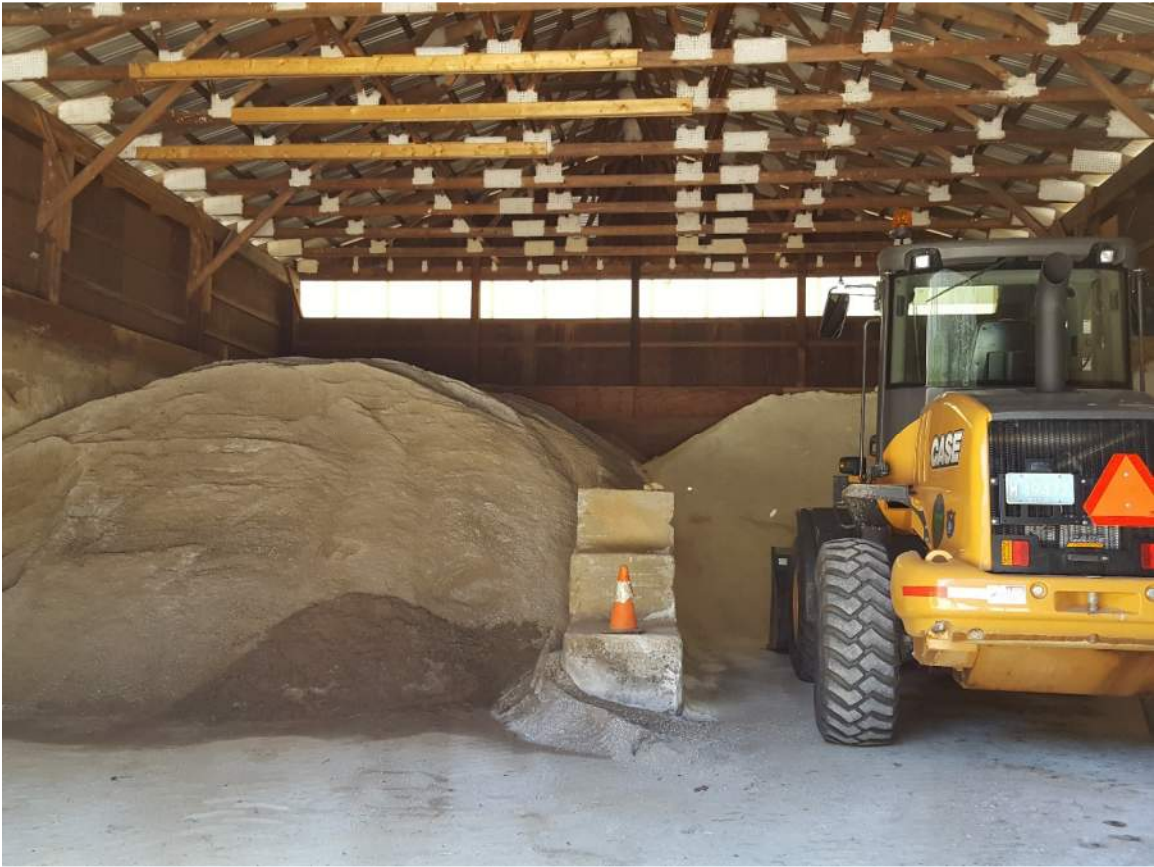
Figure 5: Forty year old Salt Shed interior bays house material and equipment.
