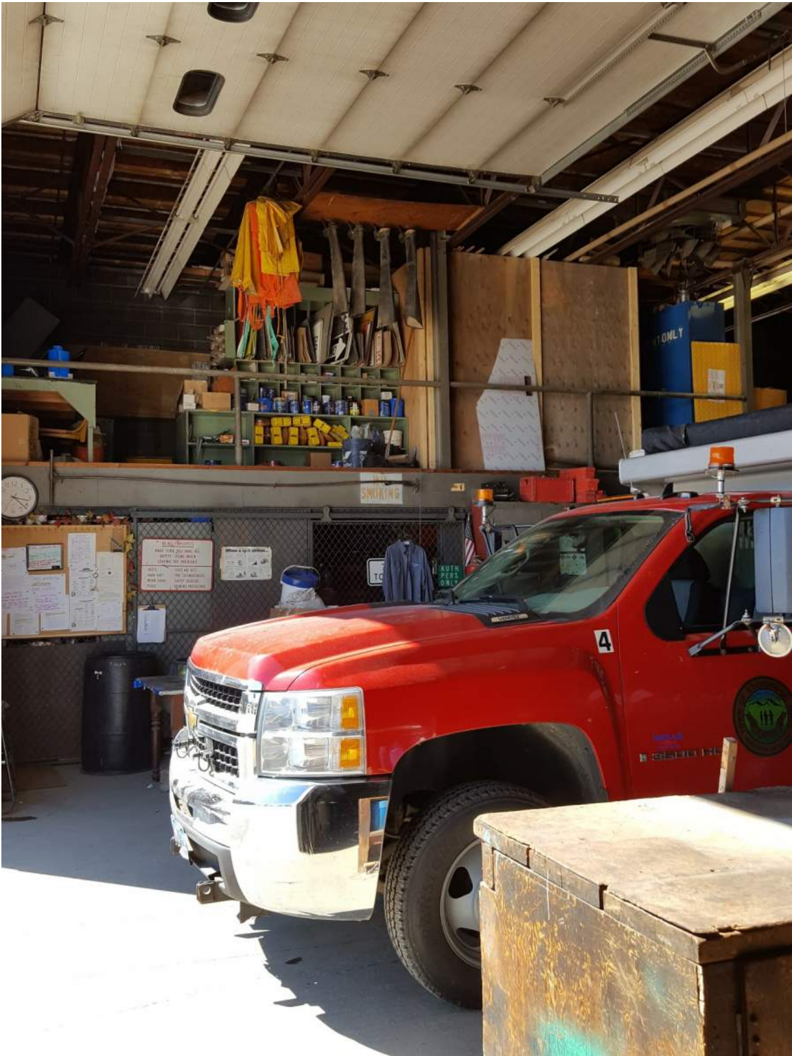
Figure 16: A secure two-story crib for specialized equipment and supplies lines a portion of the west wall.
